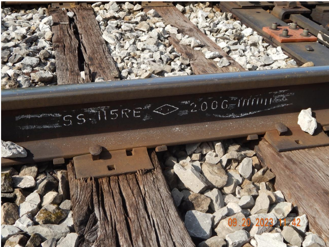
Figure 16. 115-lb Rail on CN Mainline
