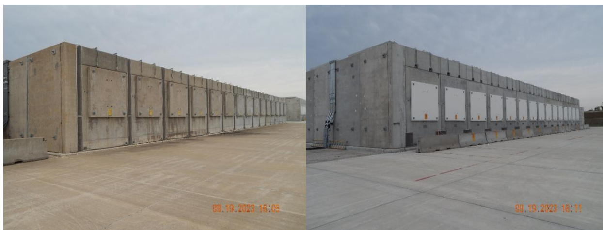
Figure 5. NUHOMS Dry Storage Systems at the Duane Arnold ISFSI
