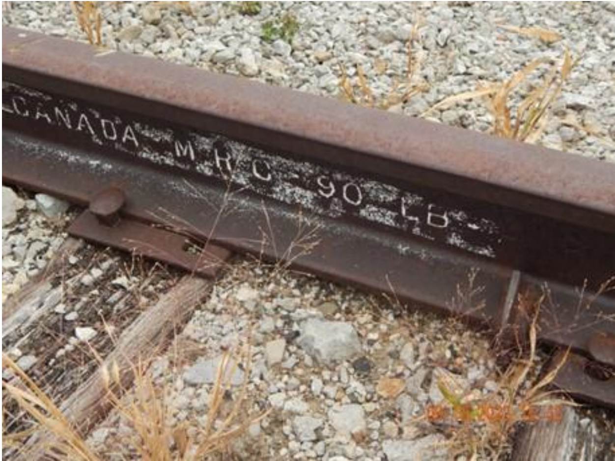
Figure 10. 90-lb Rail at Transload Locations
