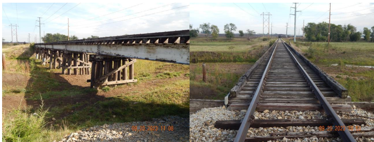
Figure 12. Trestle on Onsite Rail Spur
