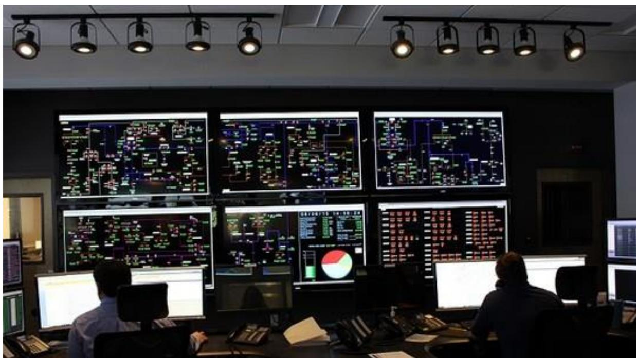
Figure 2: Modernized distribution system control room with SCADA and OMS, taken from [19].
