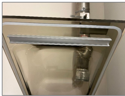
Figure 4. Seal Pad Holder
