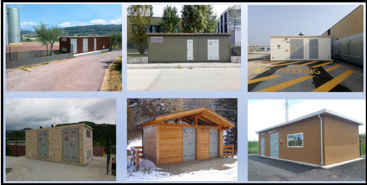
Figure 27. Examples of e-houses (pictures are courtesy of Romeo Colombara, Electric Engineer).
