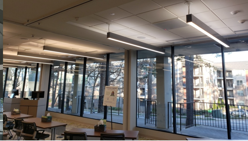
Figure 8: The group room with no partitions closed. The CCT of the pendant linear luminaires in the partitionable area on the right is higher than those of the smaller, subdividable classroom areas on the left, even though all are programmed to match in CCT and output. Photo: SimTigrate Design Lab.
