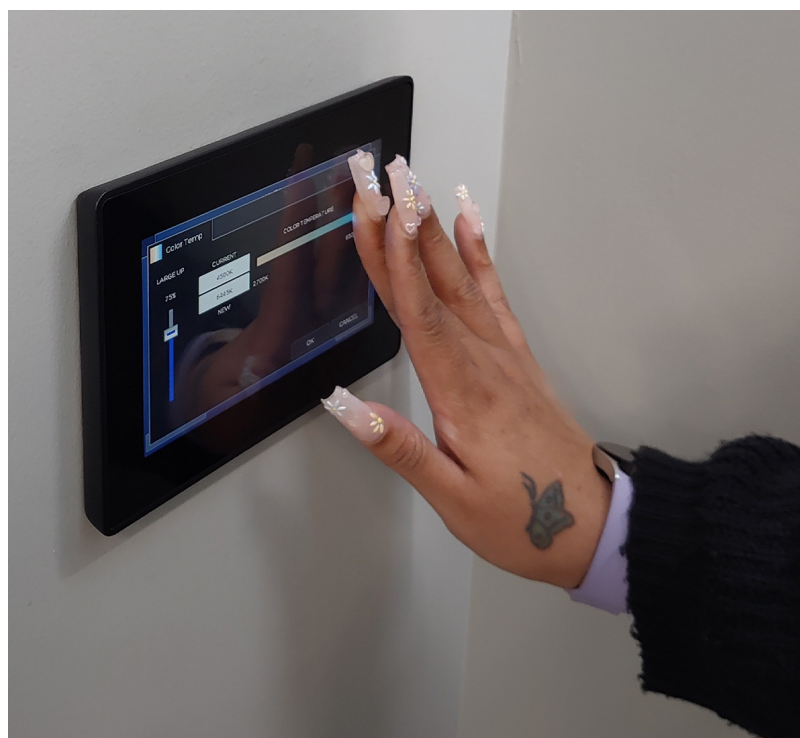
Figure 5: A staff member adjusts the lighting conditions at the touchscreen user interface. Users can adjust the intensity and CCT settings.
