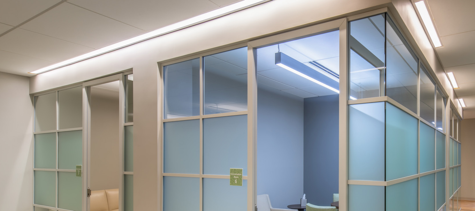
Figure 9: Tunable lighting in the consultation rooms can be adjusted to suit individual preferences and needs, although the very cool light setting here was not intentional. Photo: SimTigrate Design Lab.
