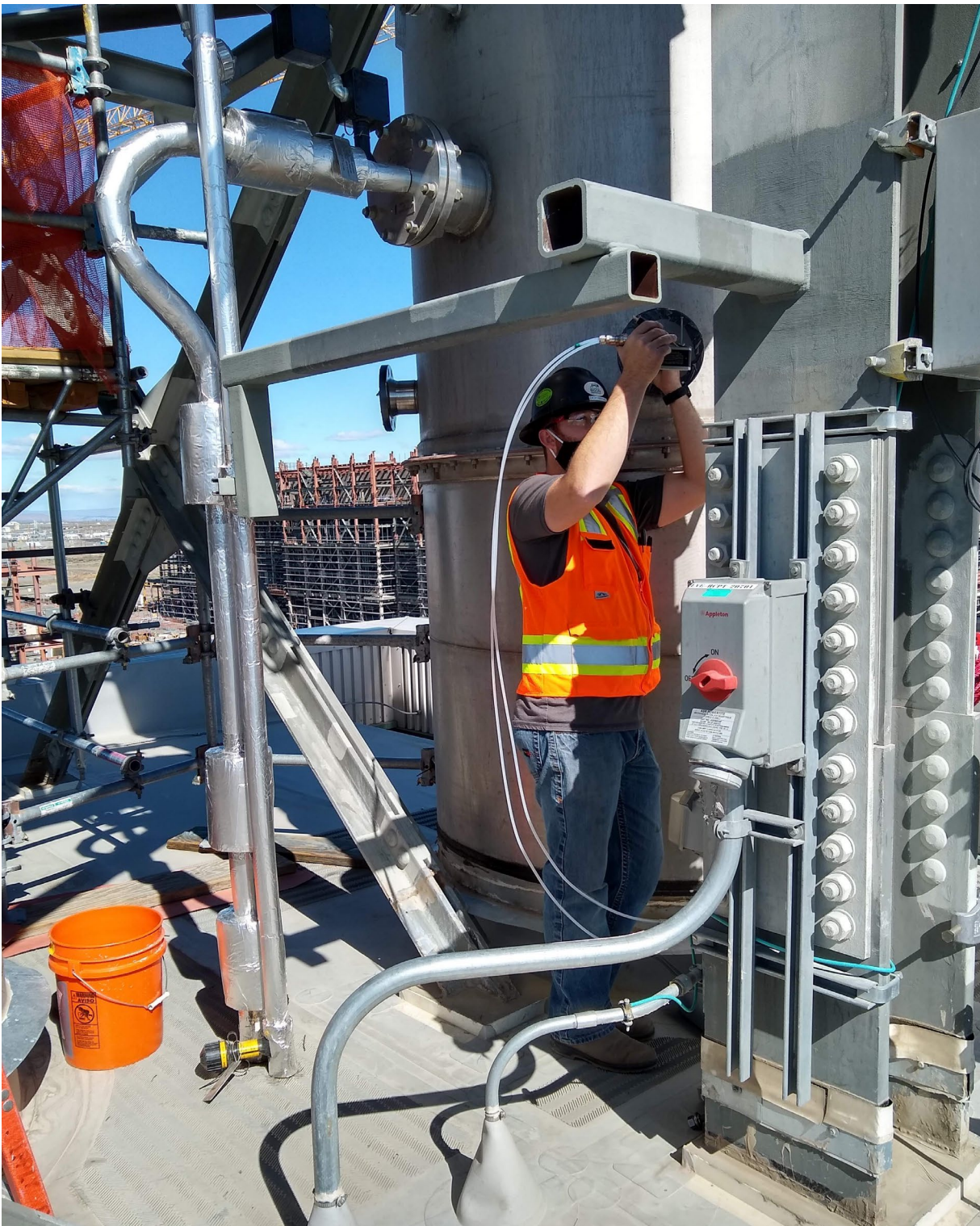
Figure 5. LAW LV-C2 Stack on the Facility Rooftop. The Bison staff member is measuring flow angle at the east port, and the west port is visible behind him.
