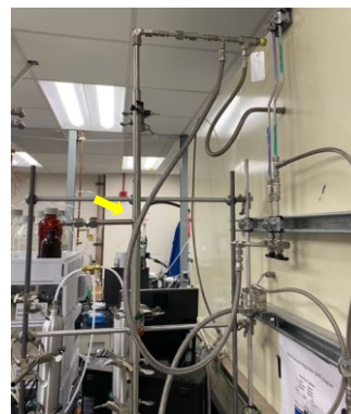
Figure 9. Photograph of separator as constructed. Arrow points at the join between the shell and the outlet.
