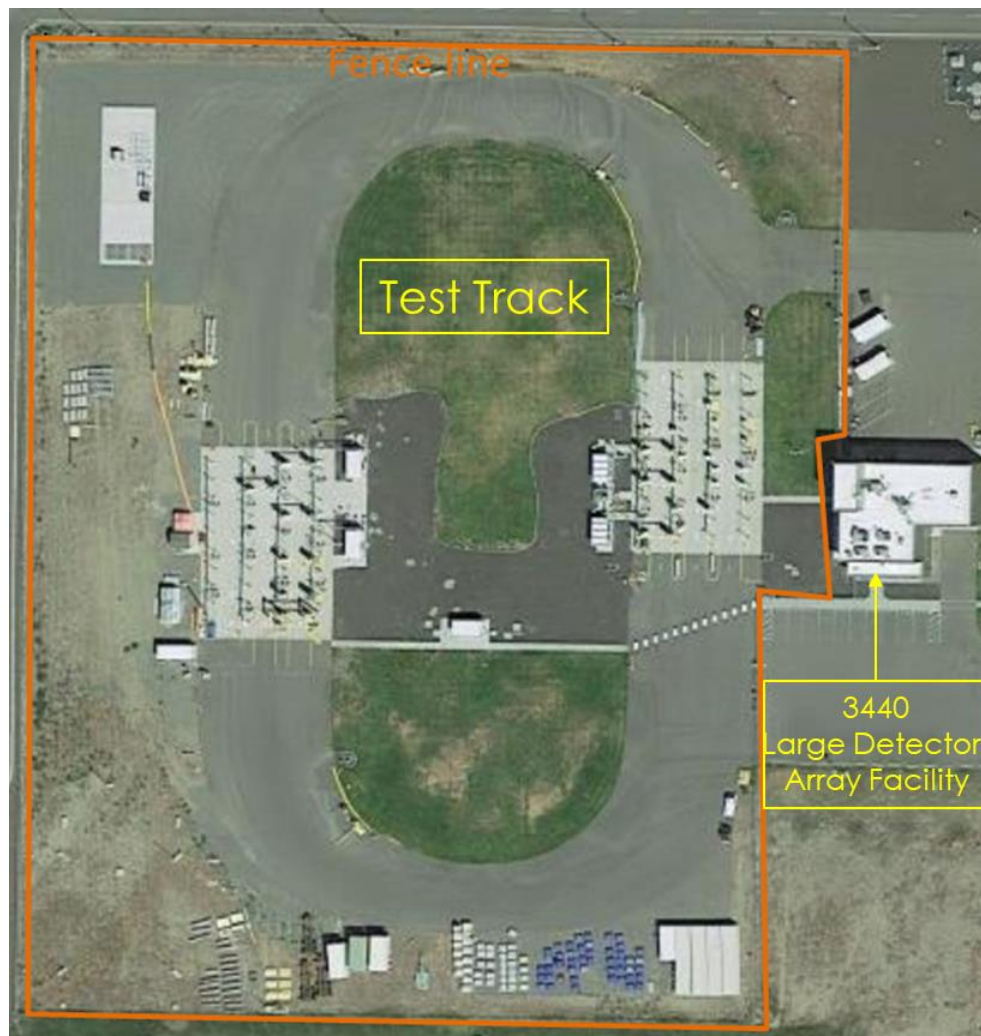
Figure 5. PNNL's 3440 Test Track Used for UAV and Human Radiological Surveys
