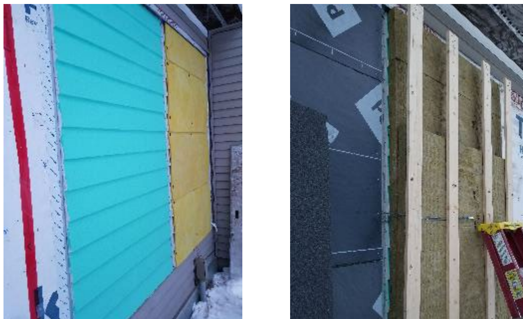
a) Liquid Applied Membrane (left, green). b) Mineral Fiber Panels and Furring Strips.
