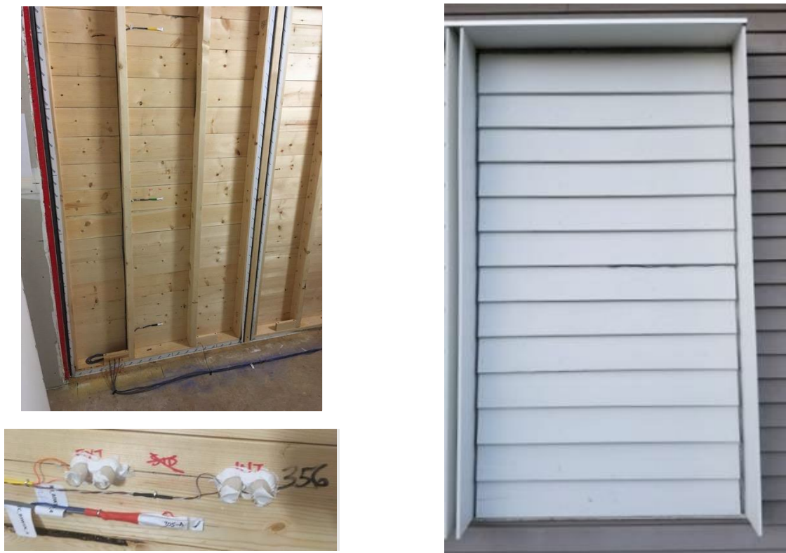
Figure 3-6 Example Sensor Installation in Wall A – Base-Case
