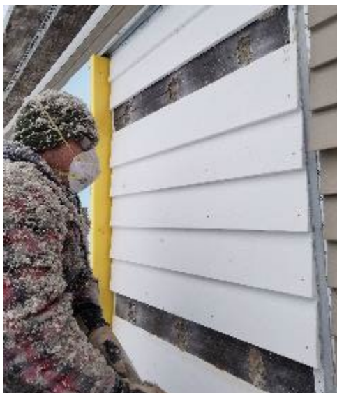
a) Cellulose insulation contractor with completed drill-and-fill, prior to hole sealing and cladding reinstall.
