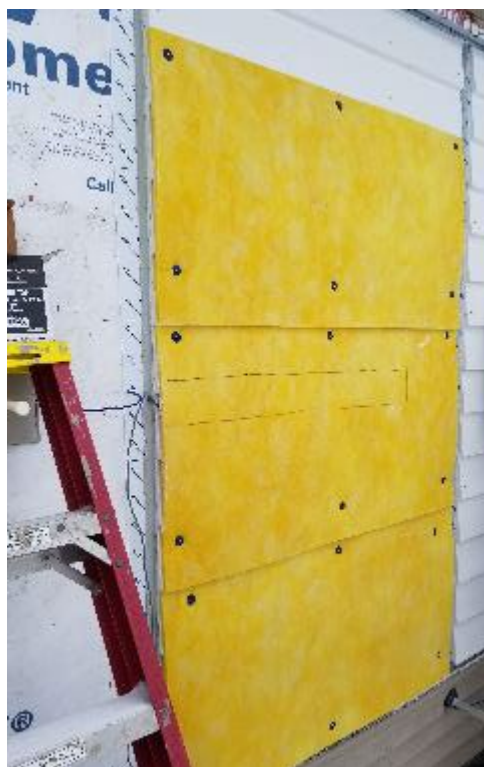
a) Interstitial Compressible Fiberglass
