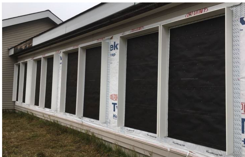
Figure 3-4 Exterior View of CRRF Test Bays Showing Baseline Wall Construction Without the Exterior Cladding Applied
