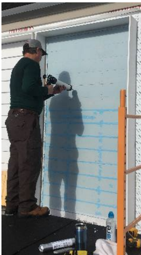
a) Caulking the Pre-Existing Sheathing.
