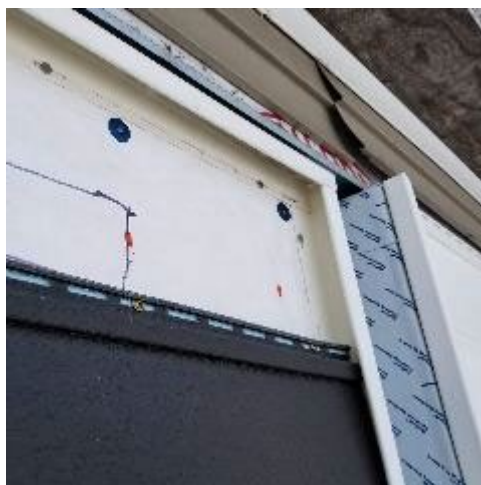
a) Close Up: VIP-Integrated Siding.
