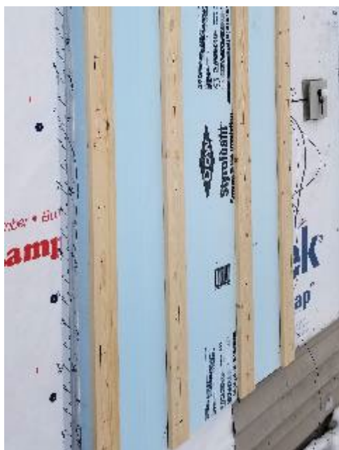
c) 2-in. XPS Layer with Furring Strips.
