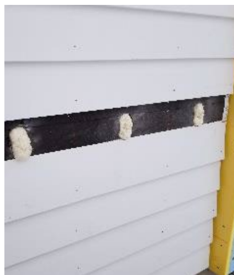
b) Holes in sheathing sealed with spray foam; foam subsequently cut flush with for siding reinstall.
