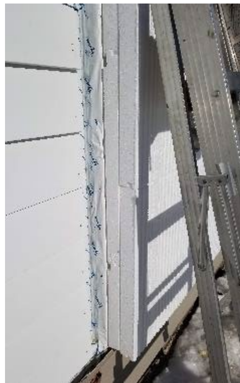
b) Installed EPS Panels
