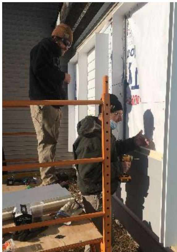
d) Installing Wall N Test Panels.
