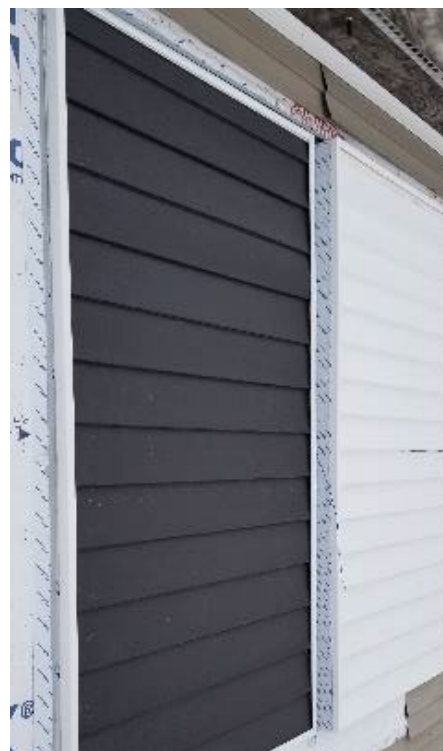
b) Installed VIP Siding
