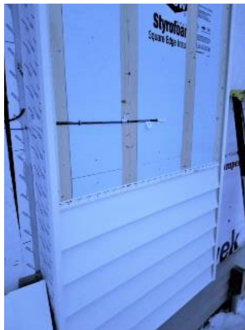
d) Backer XPS to Support Vinyl Siding.
