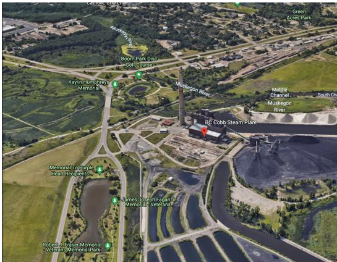
Figure 7. B.C. Cobb Generating Plant. (Source: Google Earth 2021c)
