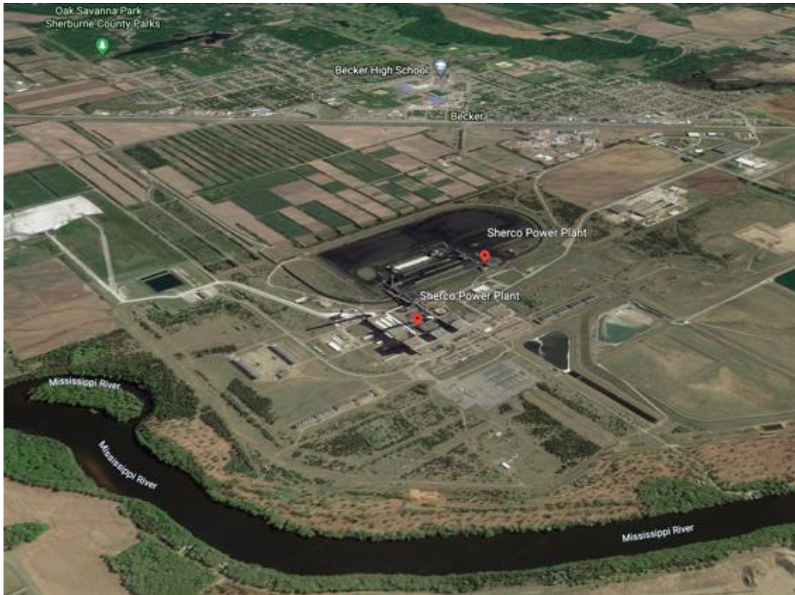
Figure 8. The Sherburne County Generating Station. (Source: Google Earth 2021d)
