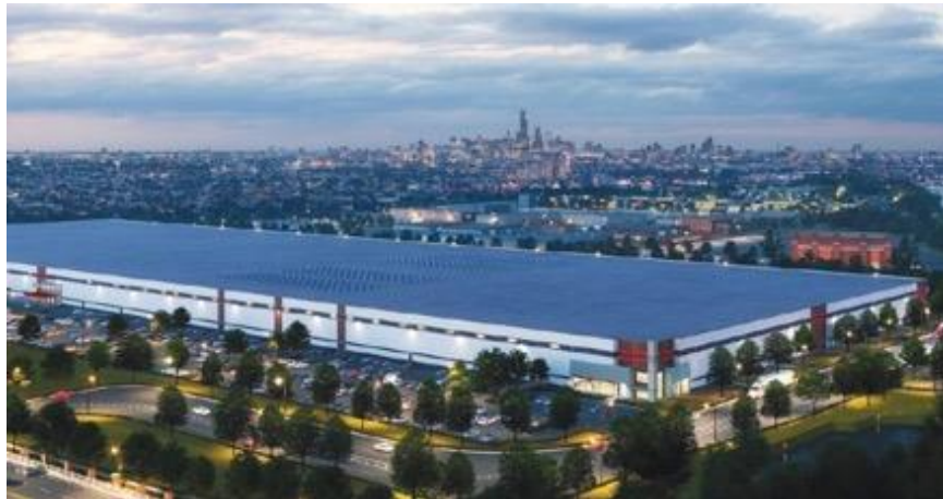
Figure 4 Named “Exchange 55,” a distribution center offers a Leadership in Energy and Environmental Design-certified warehouse building, over 1,000 jobs for the surrounding community, and accommodation of rooftop solar panels, electric vehicle charging infrastructure, and green landscaping. (Source: Exchange-55.com)
