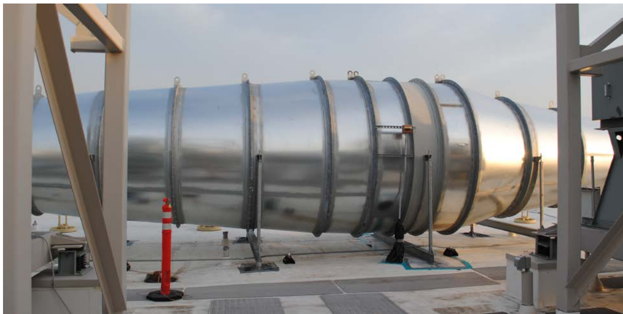
Figure 3. Photograph of Duct of the 3420 Building Exhaust System with Air Blender Installed (matte grey section with a support stanchion)
