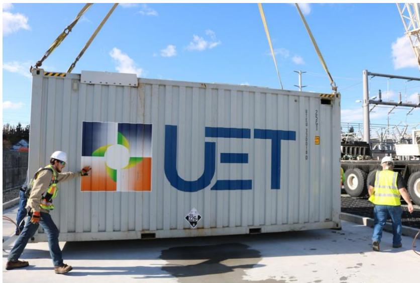
Figure 2.5. UET Vanadium Redox Flow Battery Installation in Everett, Washington
