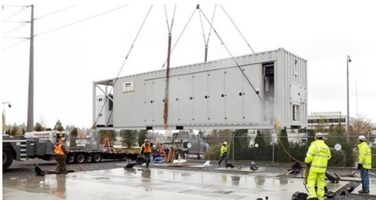
Figure 2.3. Installation of MESA 1 Battery System at Everett, WA Substation
