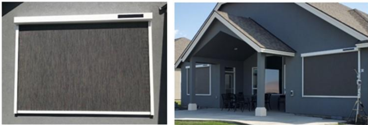
Figure 14. Exterior Shade Application at Field Site 1
