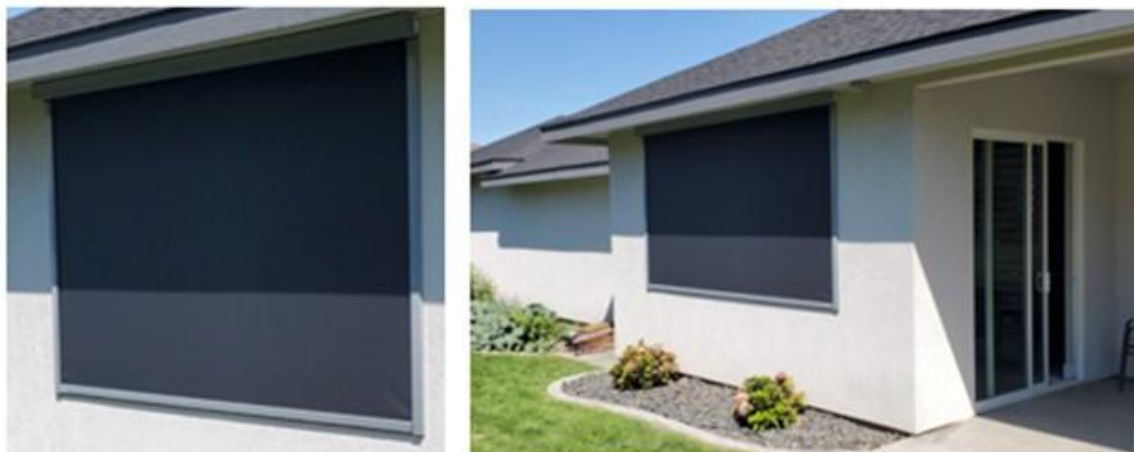
Figure 15. Exterior Shade Application at Field Site 2
