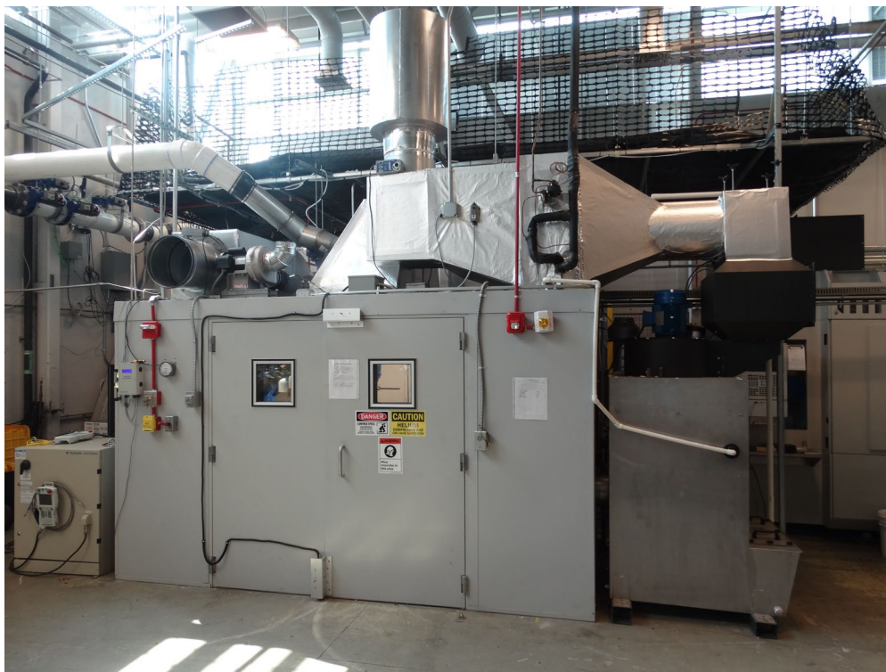
Figure 1-2 Helium recovery system installation (courtesy of ARL).
