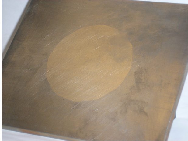
Figure 3-10 Ni CS deposit filling a blended region of simulated corrosion in a ¼ in. carbon steel plate (sample courtesy of ARL). Ni CS deposit is the brighter circular region in the center of the plate.
