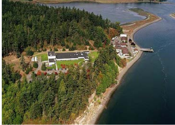
Figure 10. Aerial photograph of the PNNL's Marine Sciences Laboratory located at the mouth of Sequim Bay.
