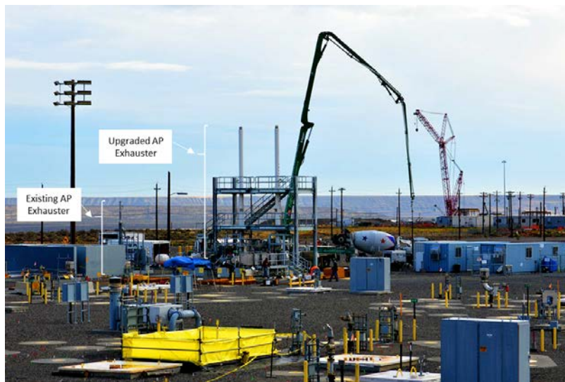
Figure 1. AP Tank Farm During Construction of the Upgraded AP Exhauster System
