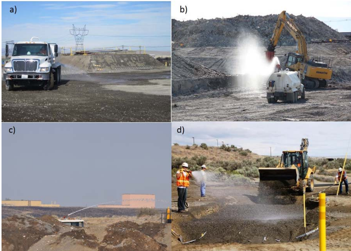
Figure 1-4. Examples of water applications to control fugitive dust at Hanford. a) Water truck applying water to ground surface at 100K b) Water truck with canon spraying water at excavator c) Water canon used for dust suppression at 618-10 Burial Ground d) Hose end sprayer used to apply water for dust control for 200W Groundwater Treatment Project ( https://www.hanford.gov/c.cfm/photogallery/tags.cfm/200%20Area/2 )
