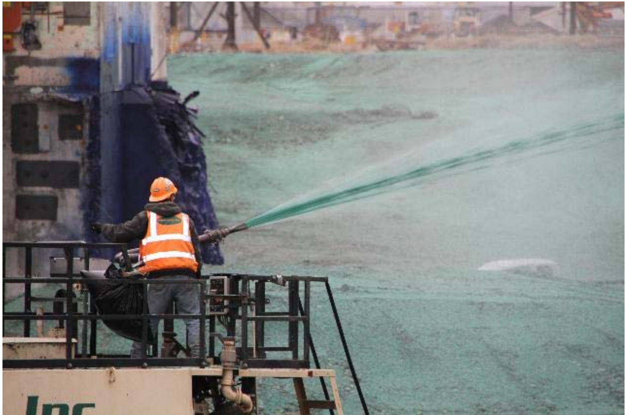
Figure A-4. Example Illustrating the Application of Hydromulch with Seeds for Revegetating Remediated Areas
