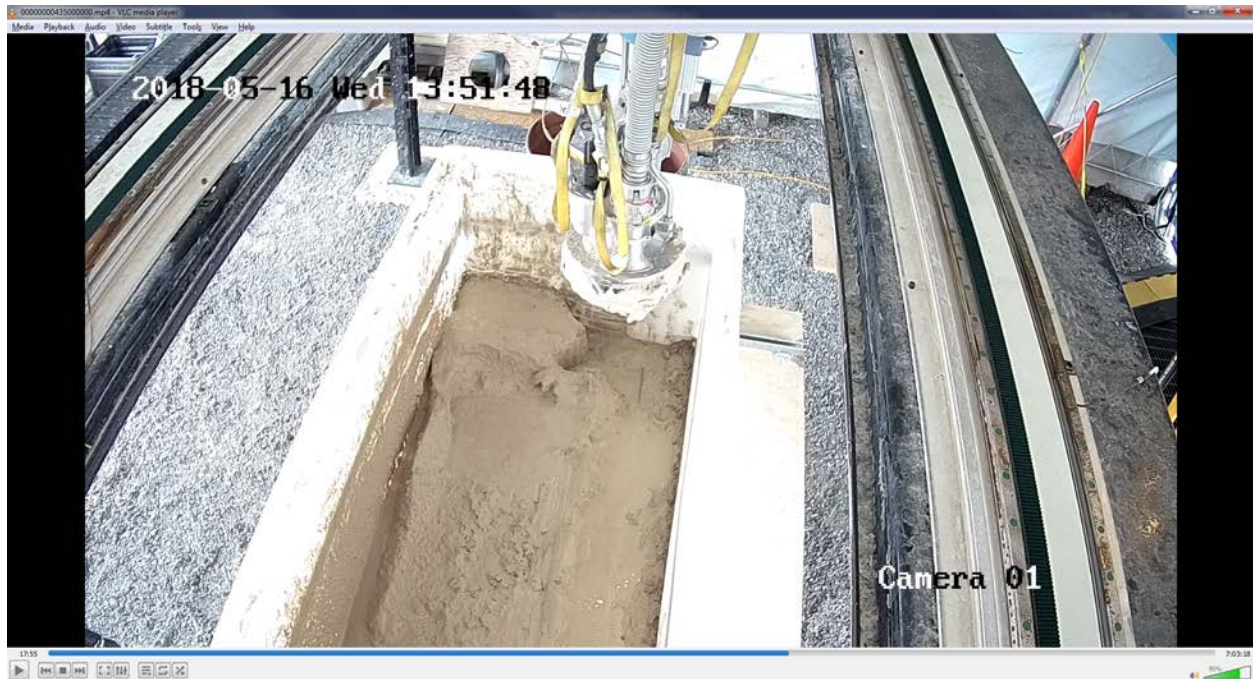
Figure TS19 – Pass 5 – Leg 3 – End (HWEE Moved – High Vertical Position)
