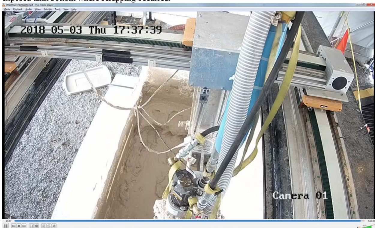
Figure LS33 - Pass 9 - Suction Clean – No flushing - Leg 3 – HWEE dragging along bottom of tank. See exposed tank bottom where scrapping occurred.
