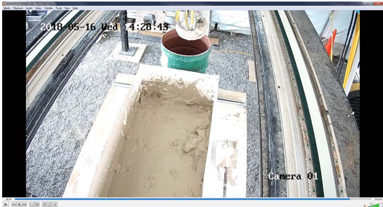
Figure TS38 – Load 4 removed.
