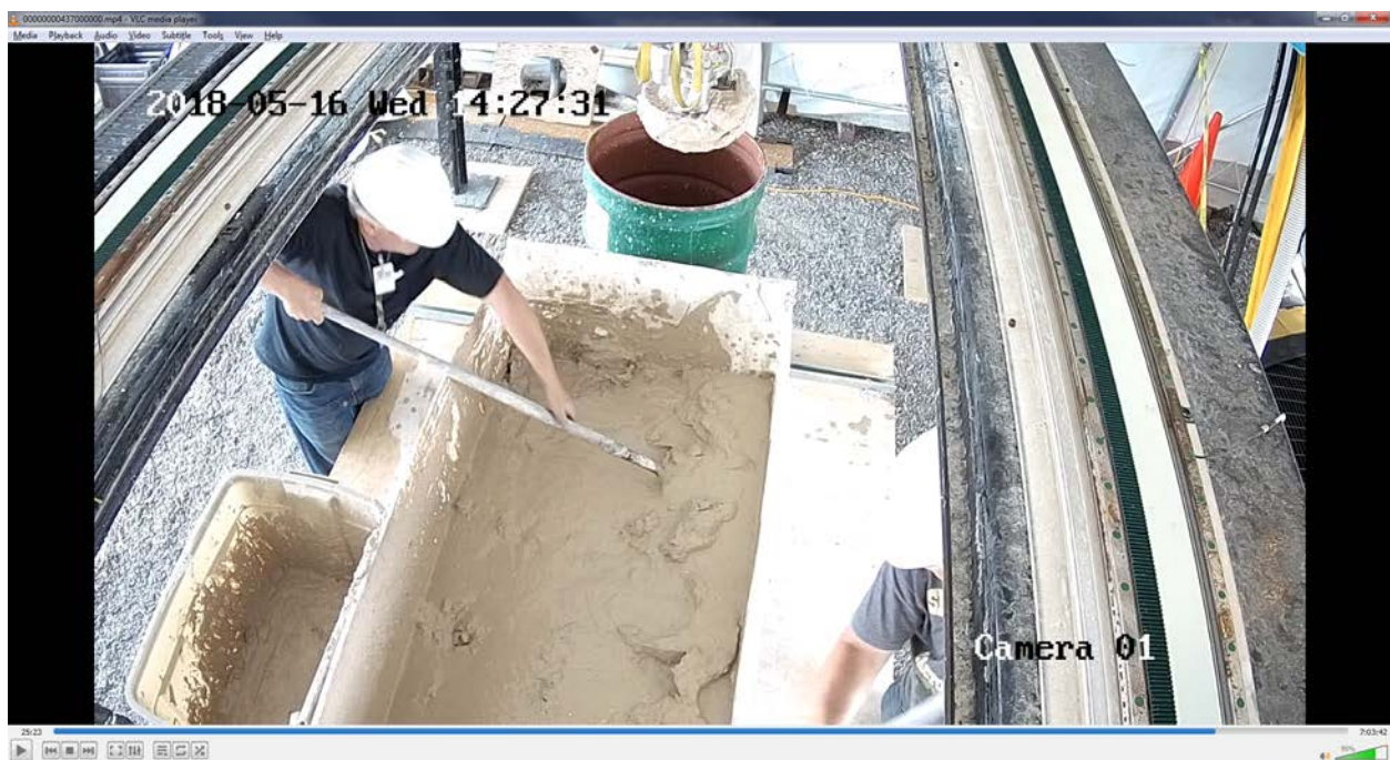
Figure TS37 – Load 4 being removed.
