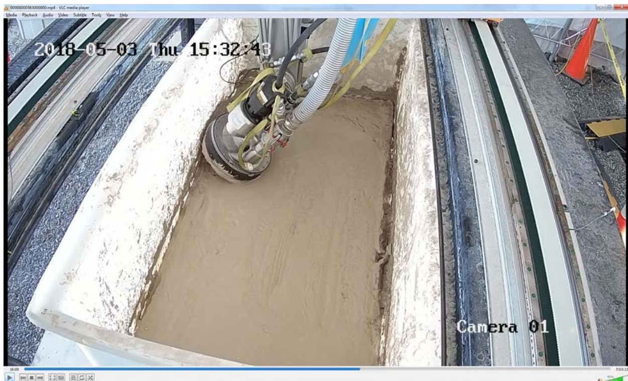
Figure LS4 - Pass 3 – Wall Cleaning - Near Side - Start
