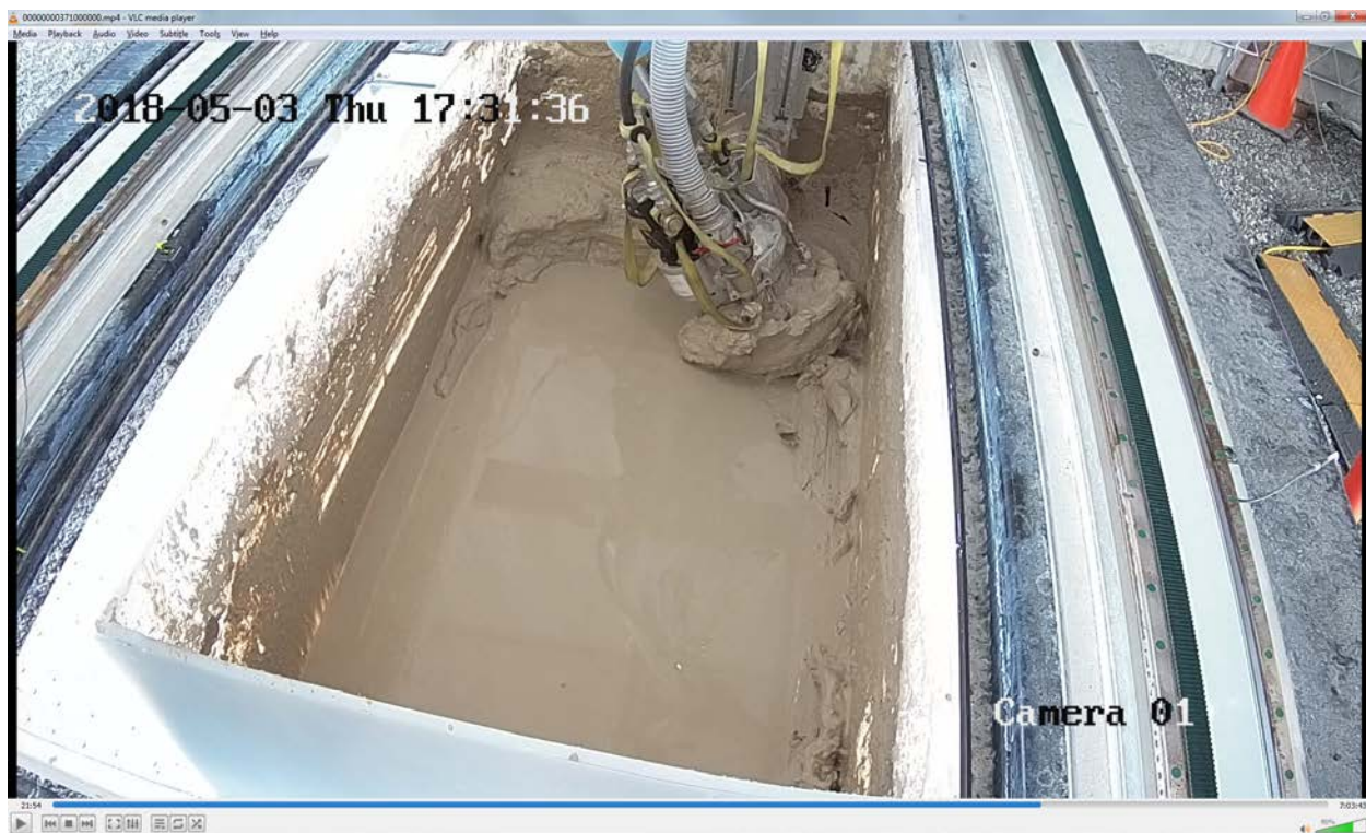
Figure LS32 - Pass 9 - Wall Cleaning - Far Side - Start
