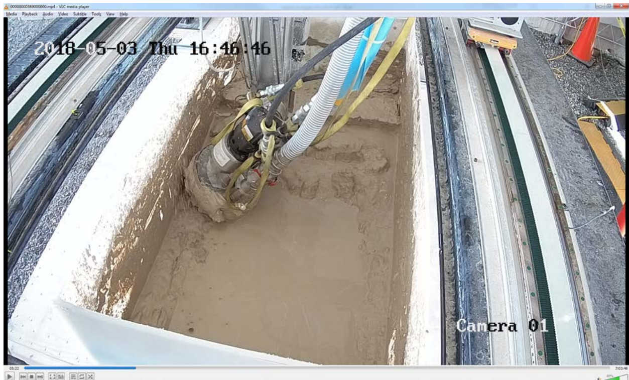
Figure LS16 - Pass 8 – Wall Cleaning - Near Side - Start
