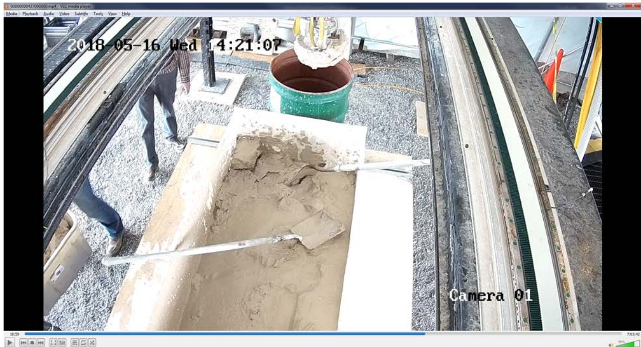
Figure TS32 – Load 1 removed
