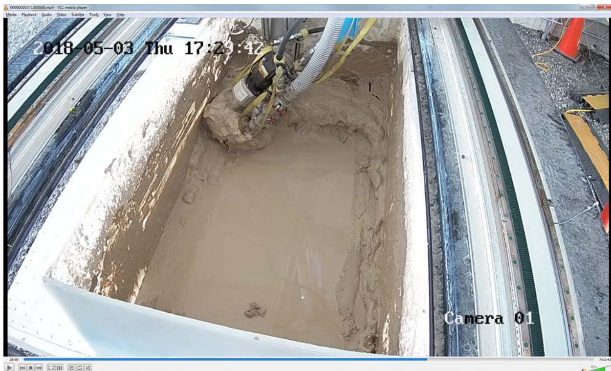
Figure LS31 - Pass 9 - Wall Cleaning - Near Side - Start
