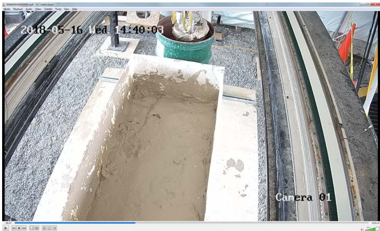
Figure TS41 – Setting HWEE pressure in Capture Tank
