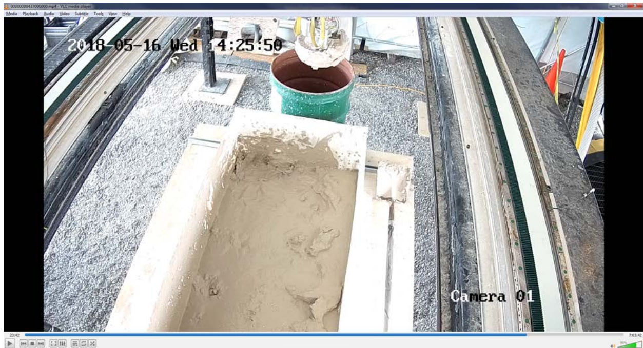
Figure TS36 – Load 3 removed.
