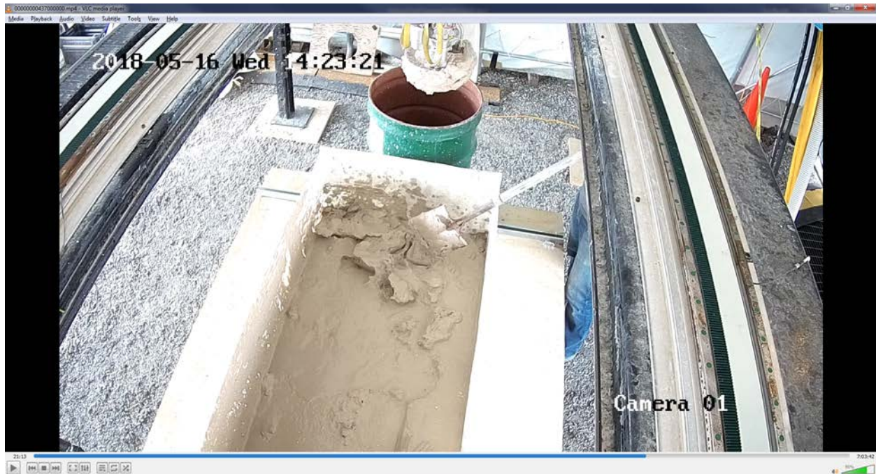
Figure TS34 – Load 2 removed.
