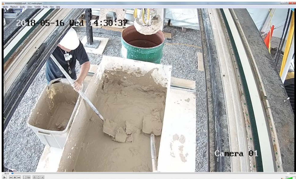
Figure TS39 – Load 5 being removed.
