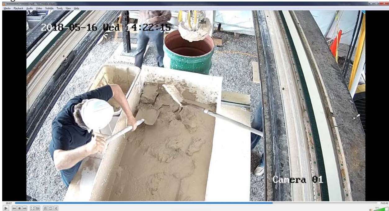
Figure TS33 – Load 2 being removed
