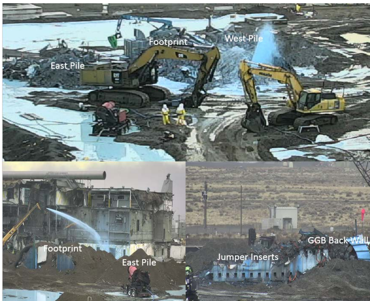
Figure A.2-1. The 236Z Building Rubble in Aerial View from the Northeast (above) Before being Covered with Soil, and from the Southeast (lower left) and from the West (lower right) after Soil Stabilization.
