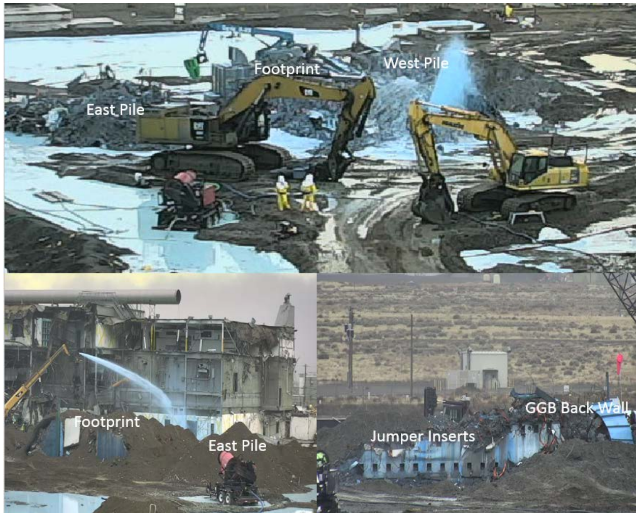
Figure 1.0-1. The 236Z Rubble Prior to Soil-Cover Stabilization in Aerial View from the Northeast (above), from the Southeast (lower left), and from the West (lower right)
