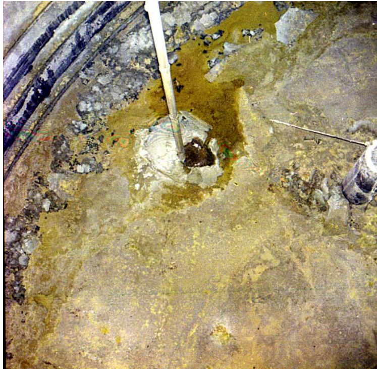
Figure 4.21. A-106 Waste Surface, Equipment Riser and ALC
