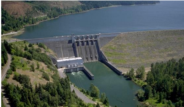
Figure 1.2. Aerial Photograph of Lookout Point Dam (courtesy of the USACE [ http://www.nwd-wc.usace.army.mil/dd/common/projects/www/pics/lop.jpg ])
