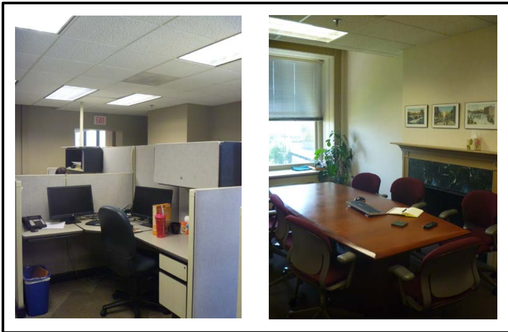
Figure 1. TeamDKB's previous offices in downtown Rochester. Open plan office (left); conference room (right). Lighting was recessed three-lamp fluorescent troffers with deep-cell parabolic louvers. Lamps were F28T8/741 fluorescent with correlated color temperature (CCT) of 3797 K, color rendering index (CRI) of 81, and an R9 of 6. Photos: Pacific Northwest National Laboratory (PNNL).
