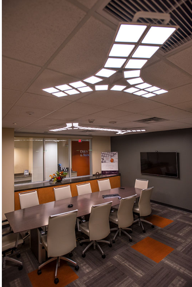
Figure 6. TeamDKB large conference room showing the 24-panel and 56-panel Acuity Brands Winona® Trilia™ configurations, plus two single panel Birot Zhen pendants over the lower cabinets at the window wall. Photo courtesy OLEDWorks LLC and DeJoy Knauf & Blood, LLP.
