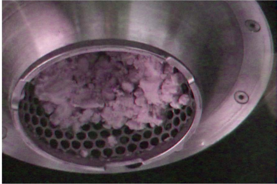
Figure 2.2. Screen Clogging during Prior Tests
