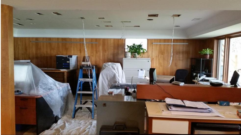
**Figure 5.** Office ceiling during construction, showing holes for fishing wires as well as precise mounting locations for the Trilia™ sections. (Photo: Leslie North.)
