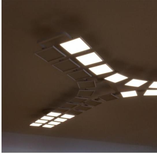
**Figure 7.** Failure of half the panels in the 24-panel triangular assembly, indicating one of the two drivers for this assembly had failed. (Photo: Leslie North.)
