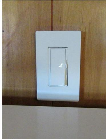
**Figure 4.** A 0-10 V dimmer installed to control output of the Trilia OLED system. (Photo: Leslie North.)
