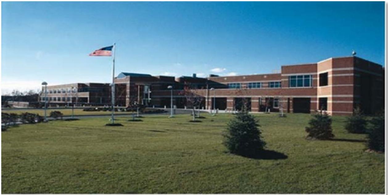
Figure 10. Exterior Photo of Philadelphia VA Facility
