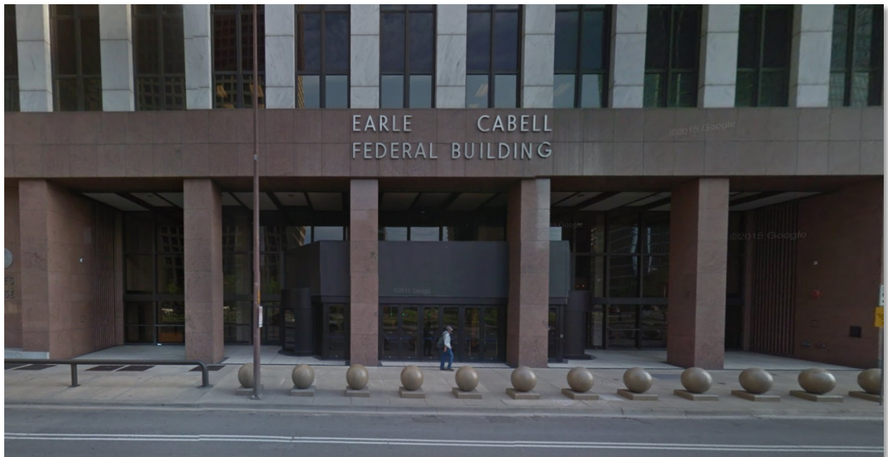
Figure 9. Exterior Photo of Cabell Federal Building
