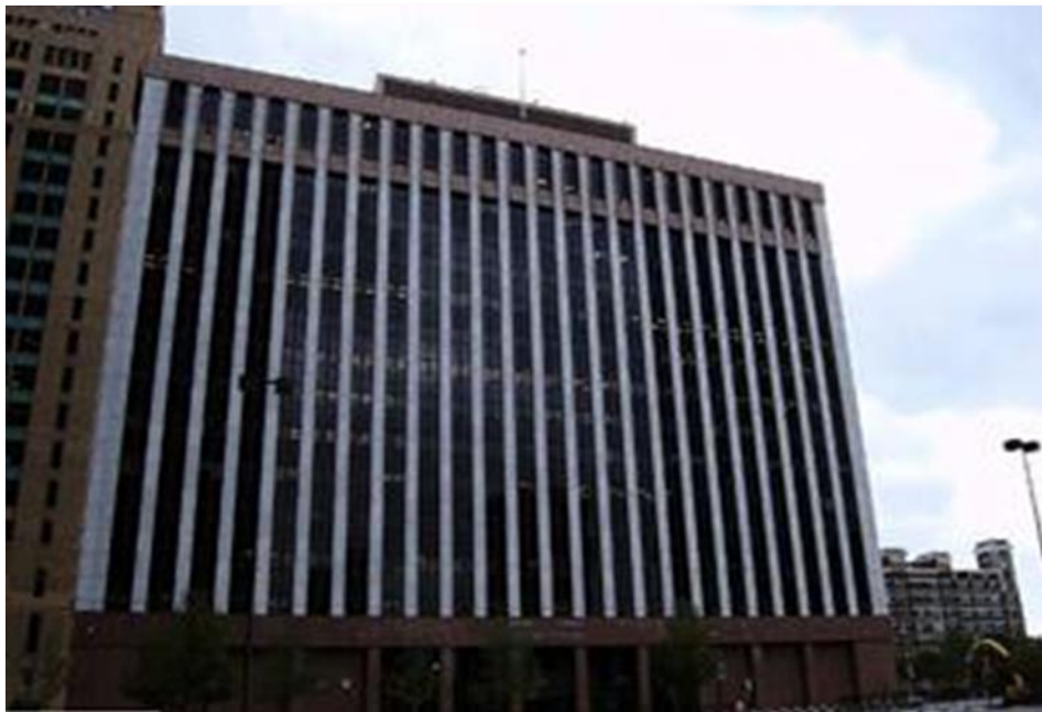
CABELL FEDERAL BUILDING (7TH FLOOR) – DALLAS, TX
