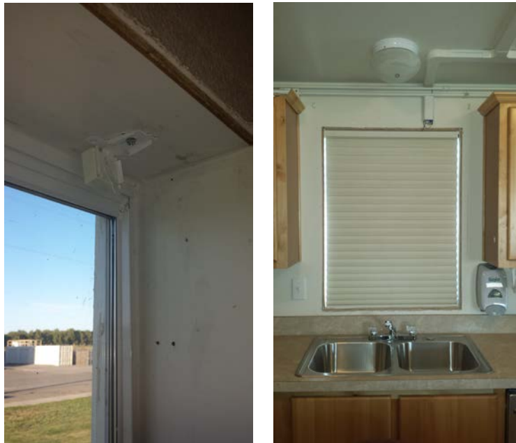
Figure 3.2. Mounting Bracket for the Cellular Shades and Example of Installed Hunter Douglas Cellular Shade
