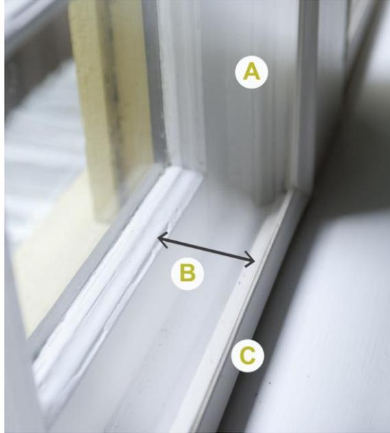
**Figure 2.2.** Indow Windows’ interior storm window insert showing the (A) acrylic window; (B) air gap between window and insert; and (C) silicone frame.
