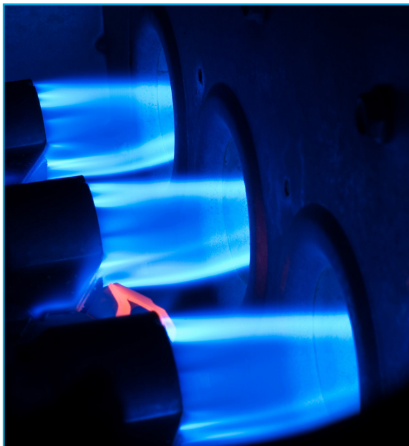
Figure 6.11. Heating chamber inside a gas furnace.
