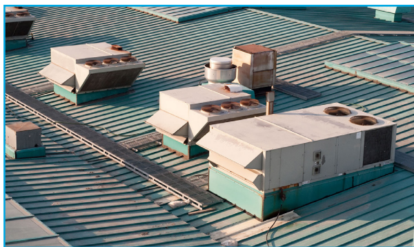
Figure 6.7. Example of several packaged rooftop units.
