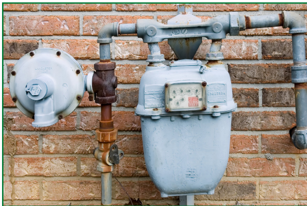
Figure 9.2. Natural gas meter.
