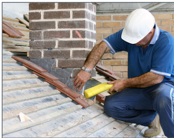
Figure 4.4. Installation of roof curb around a chimney.
