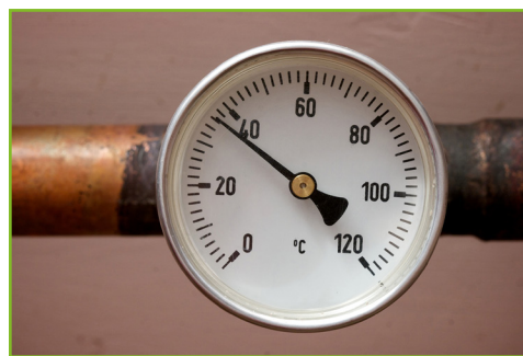
Figure 8.5. Water temperature controls and thermometer on an intake pipe.
