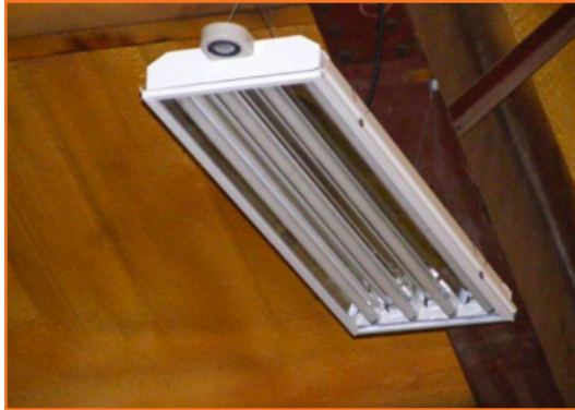
Figure 7.2. An example of a linear fluorescent fixture using only reflectors to direct light (left) and a recessed light fixture using diffusers to spread light (Image Sources [left] Courtesy of Clean Energy Resources Team; [right] PNNL).
