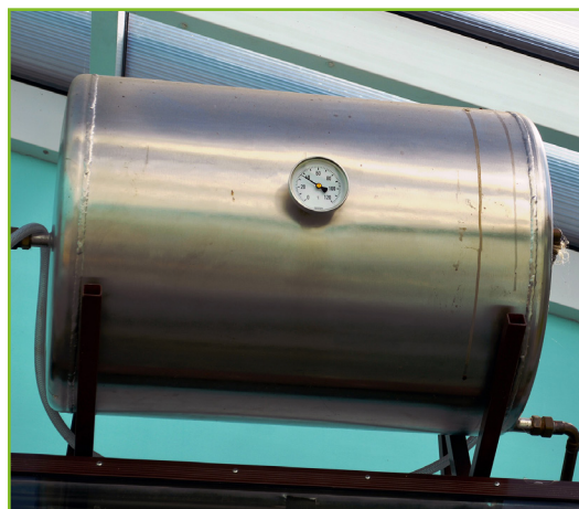
Figure 8.3. Solar panels and storage tank associated with a solar water-heating system.
