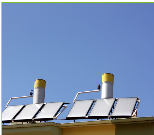
Figure 8.3. Solar panels and storage tank associated with a solar water-heating system.
