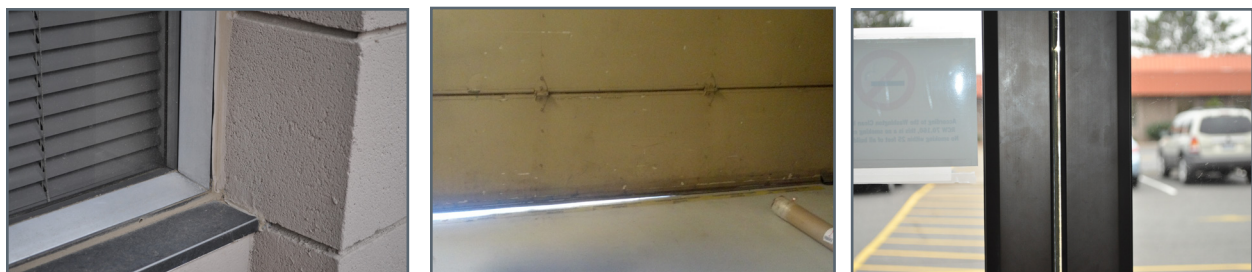
Figure 4.6. Left: caulking on exterior of building between wall and window joints. Middle: bottom of roll-up door is not properly sealed. Right: weather stripping between the double doors is missing on the right door; the lack of a tight seal creates an air gap.
