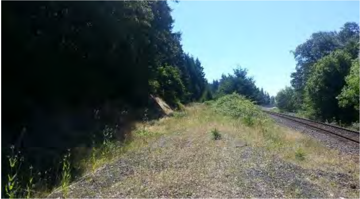
Figure 2-110. Former Trojan Rail Spur Railbed (2013)
