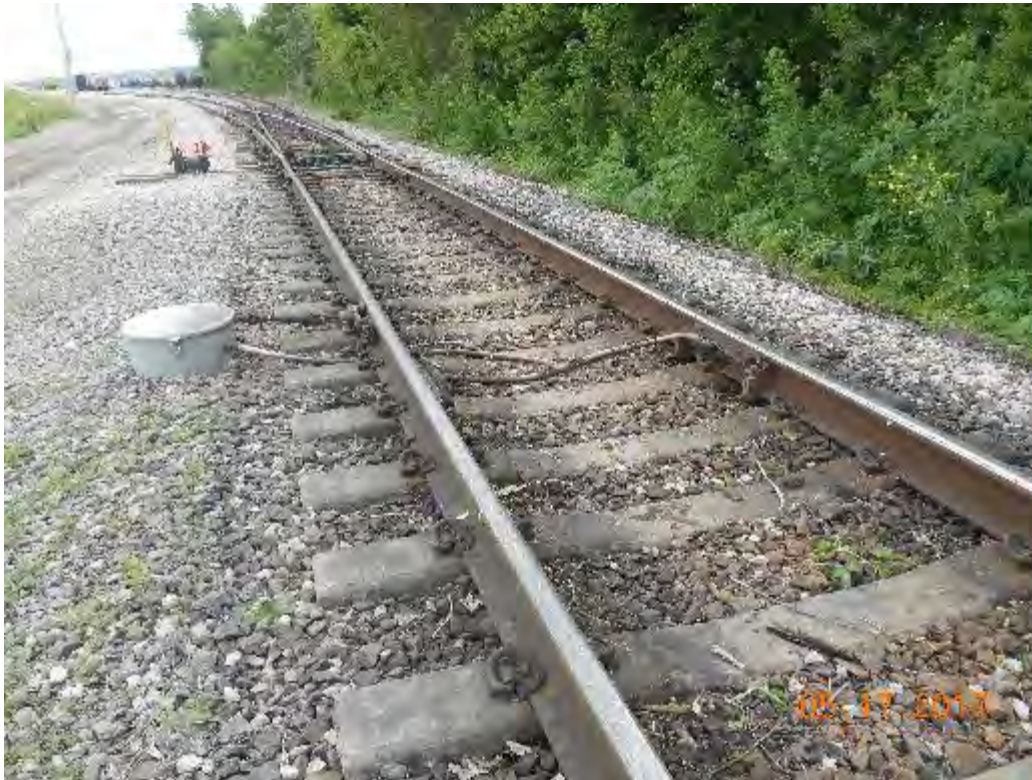
Figure 2-350. Derailer and Greaser on Cargill Industrial Spur (2017)
