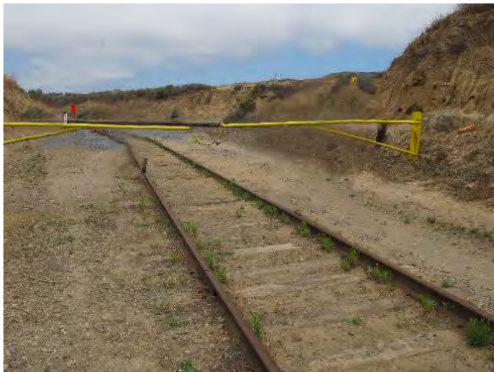
Figure B-58. Locked Facility Gate (2015)
