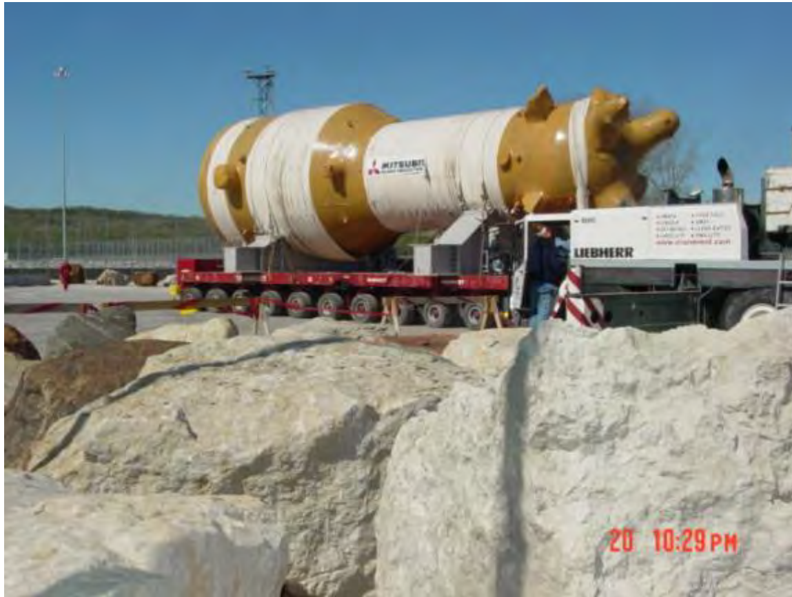
Figure 2-370. Steam Generator on Transporter After Unloading (2006)
