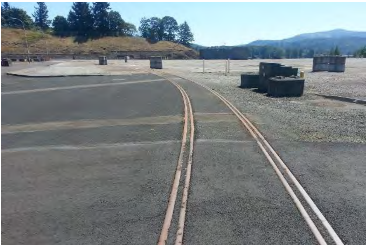
Figure 2-111. Remnants of On-site Rail Spur at Trojan (2013)
