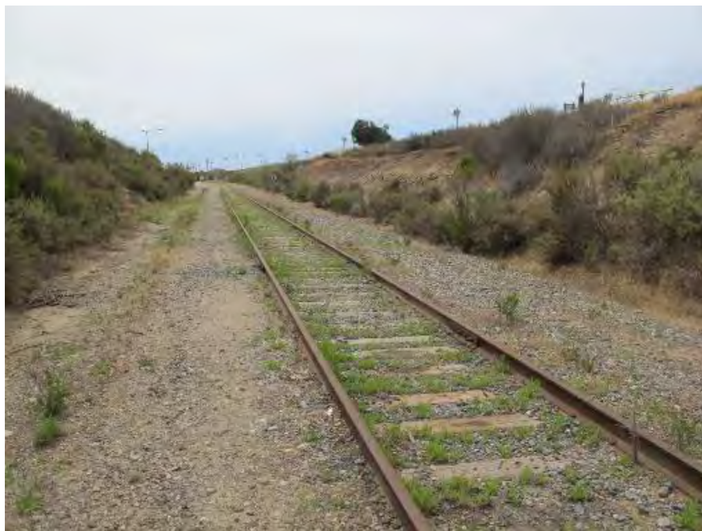
Figure 2-284. Onsite Rail Spur at San Onofre Site (2015)
