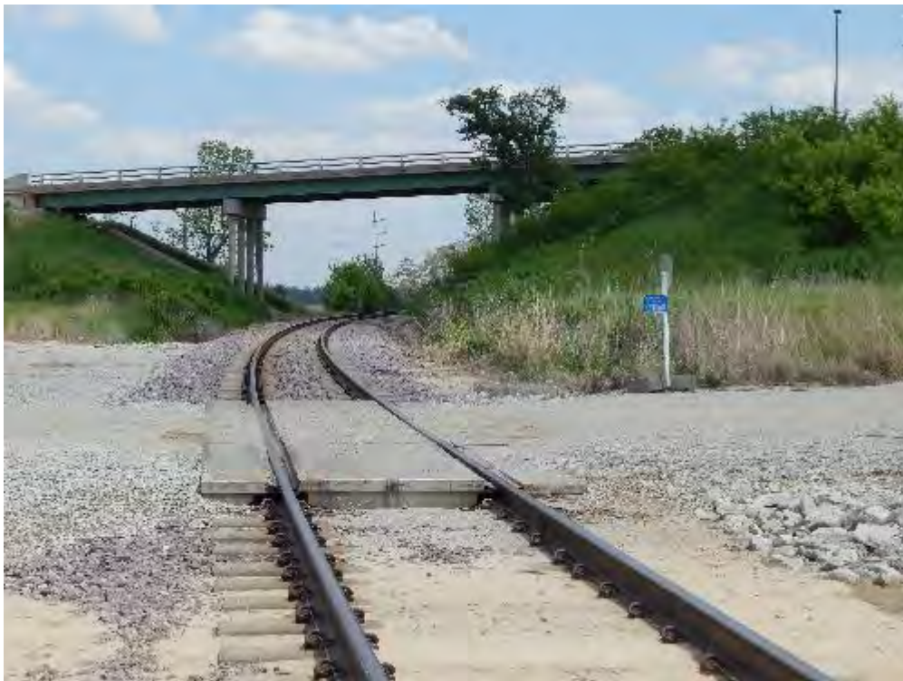
Figure 2-342. Cargill Industrial Spur (Looking Southeast) (2017)
