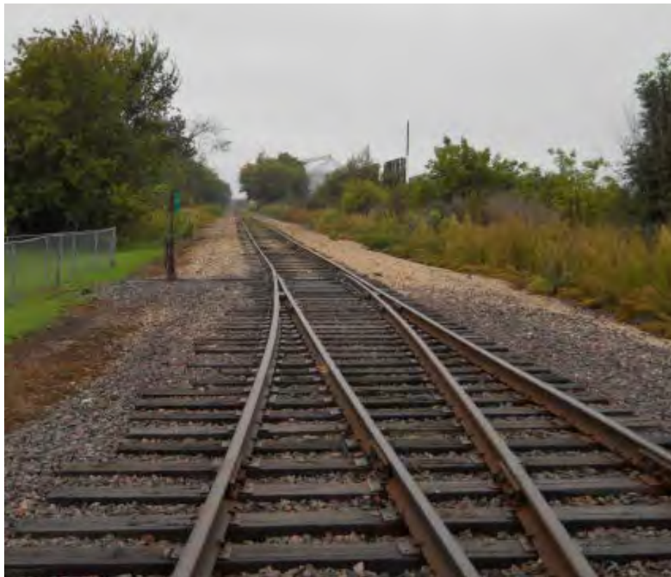
Figure B-43. Switch at Luxemburg (2014)
