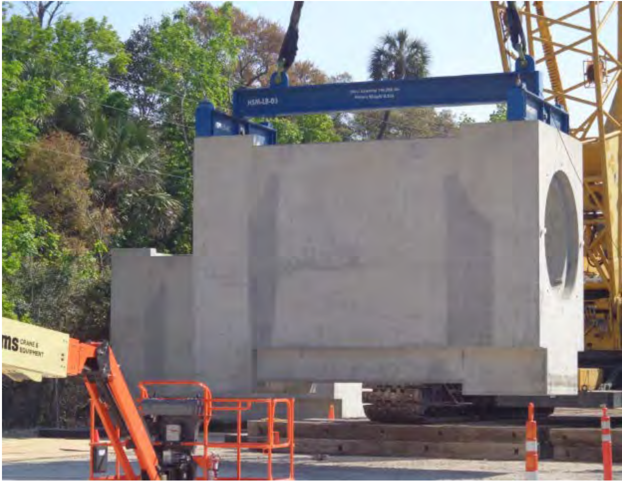
Figure 2-188. Horizontal Storage Module Being Unloaded from Railcar (2015)
