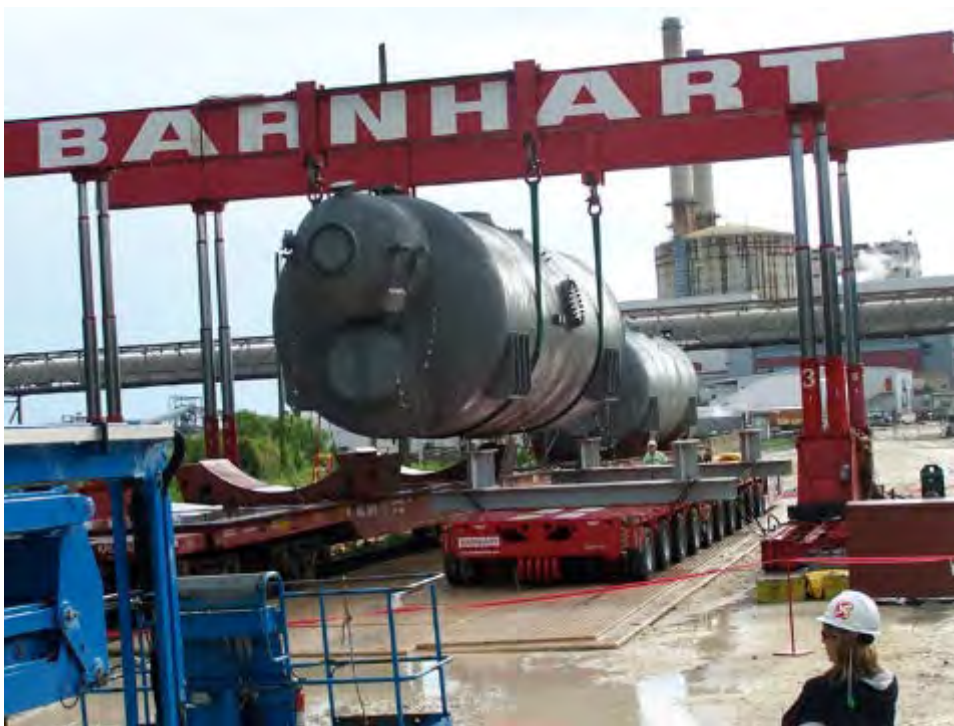
Figure 2-181. Moisture Separator Reheaters Being Unloaded at the Crystal River Site (2009)
