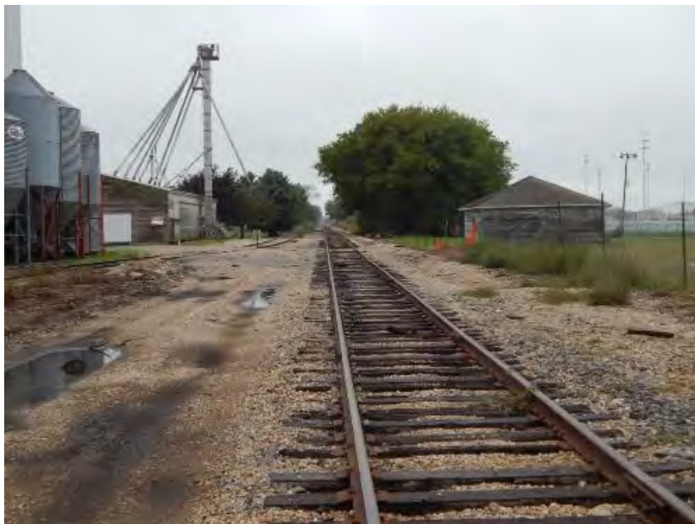
Figure 2-211. Potential Luxemburg Transload Location (Looking West) (2014)
