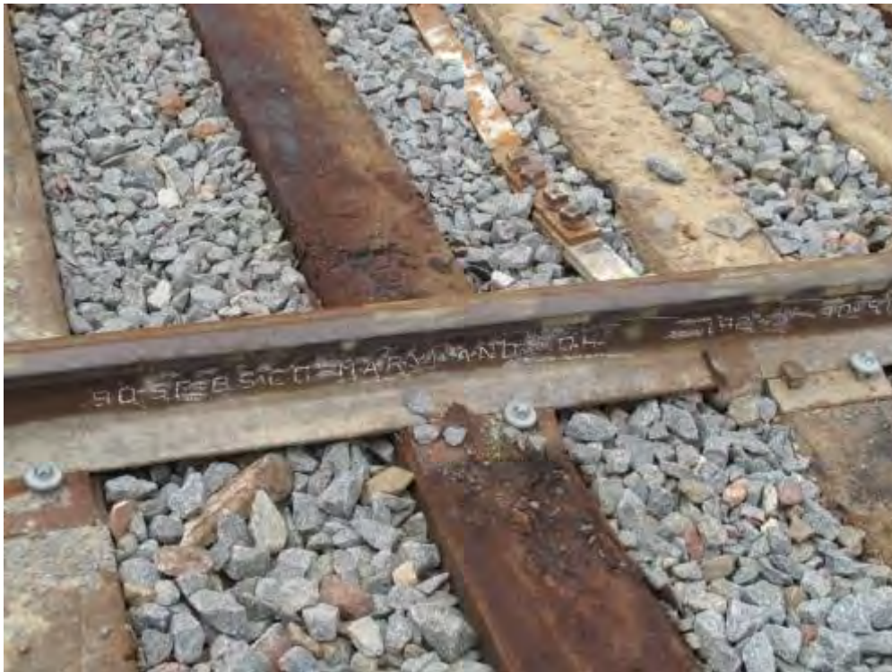
Figure B-60. Site Lead 90-lb. Rail (2015)
