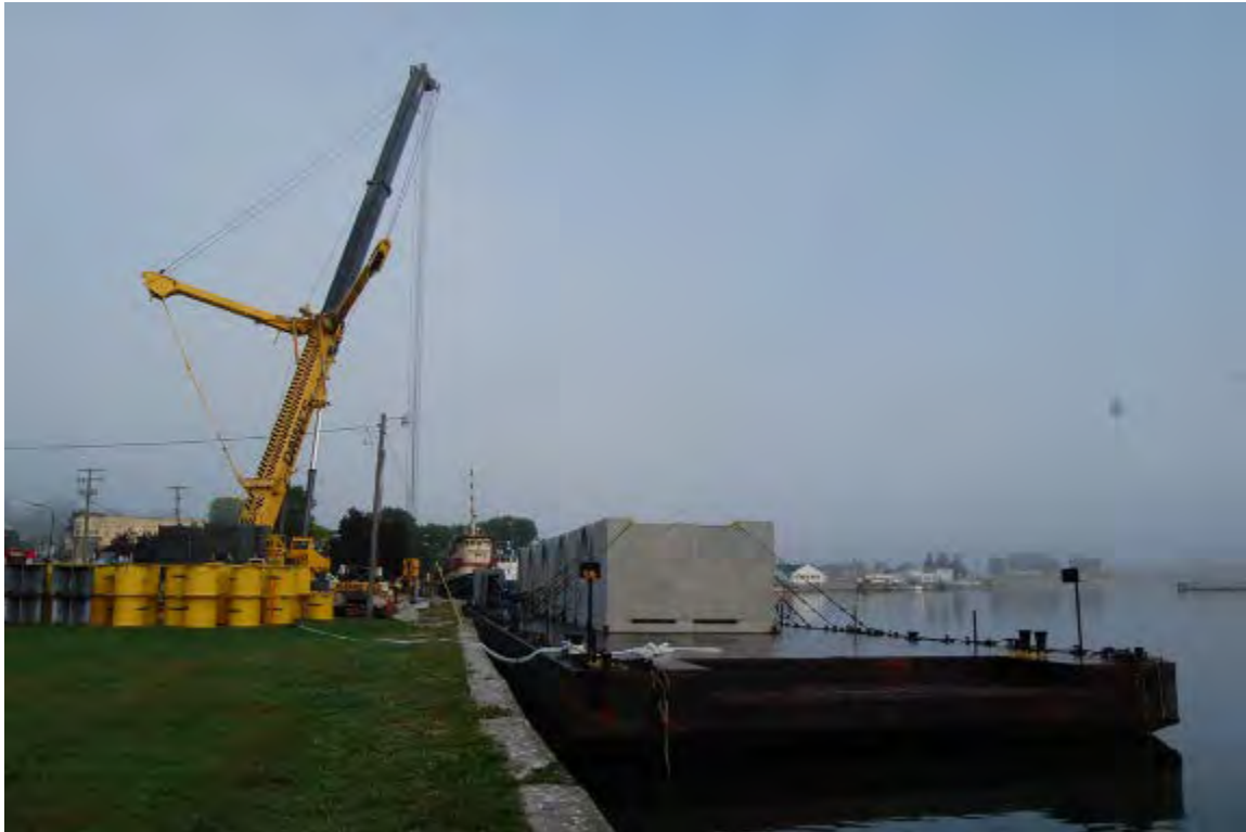
Figure 2-251. Horizontal Storage Modules Being Unloaded from a Barge (2013)
