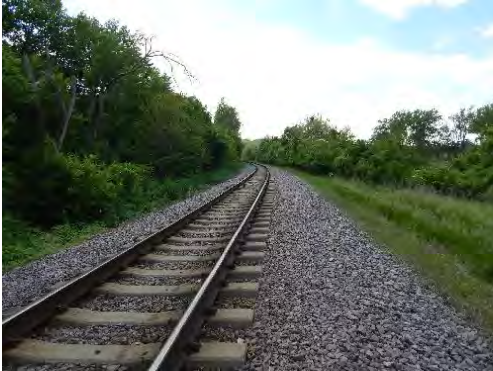
Figure 2-341. Cargill Industrial Spur (Looking Northwest) (2017)
