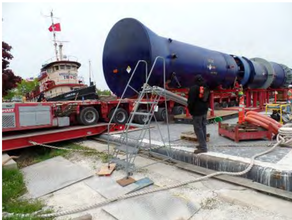
Figure 2-256. Fourth Steam Generator Moving onto Barge (2014)
