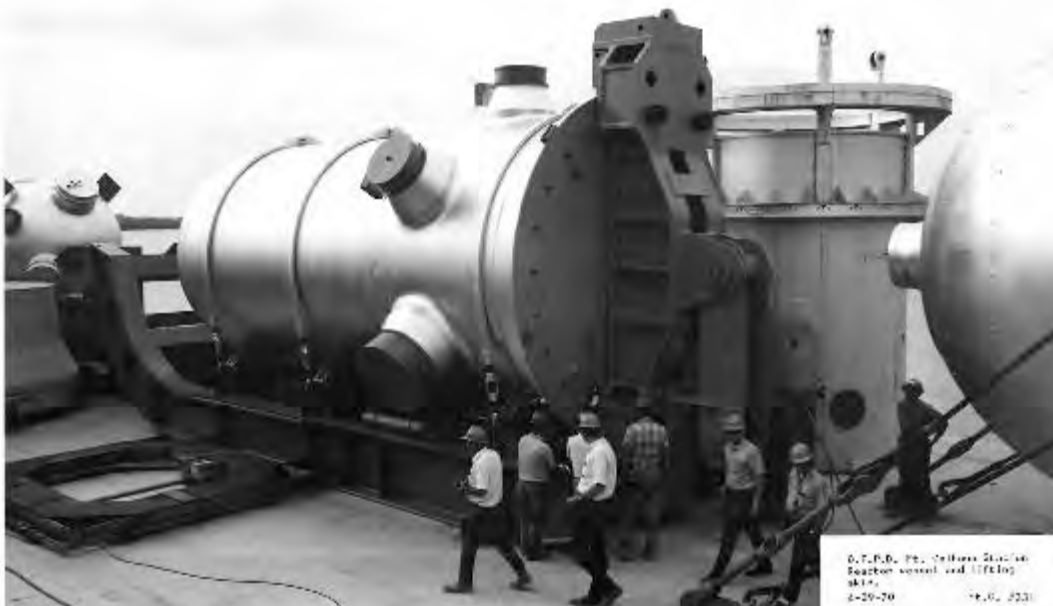
Photo courtesy of Fort Calhoun
