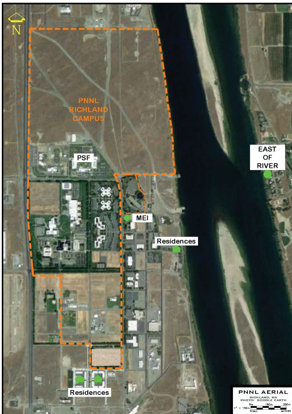
Figure 3.1. Locations of PNNL Richland Campus Potential Receptors
