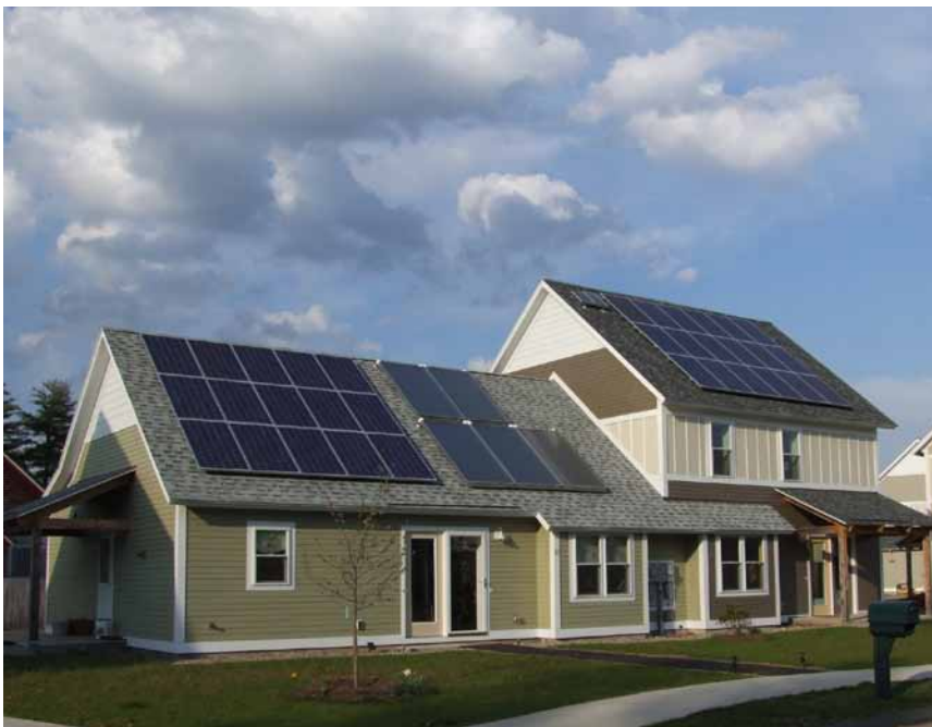
Both photovoltaic and solar thermal water heating panels are mounted on the roof of this duplex in the Wisdom Way Solar Village, an affordable housing project in western Massachusetts built by Rural Development, Inc. with design assistance from the Consortium for Advanced Residential Buildings (CARB), a Building America research team (Photo source: Steven Winter Associates).
