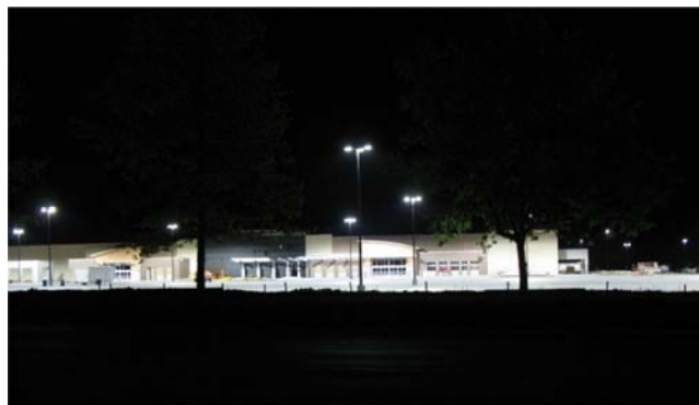
Figure 2.9. Façade during construction
