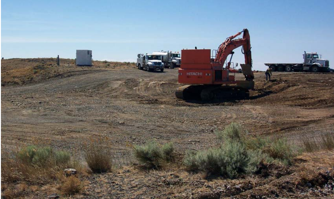
Figure 2.8. Unit 4: Area to be Revegetated where 6652-C Buildings were Removed
