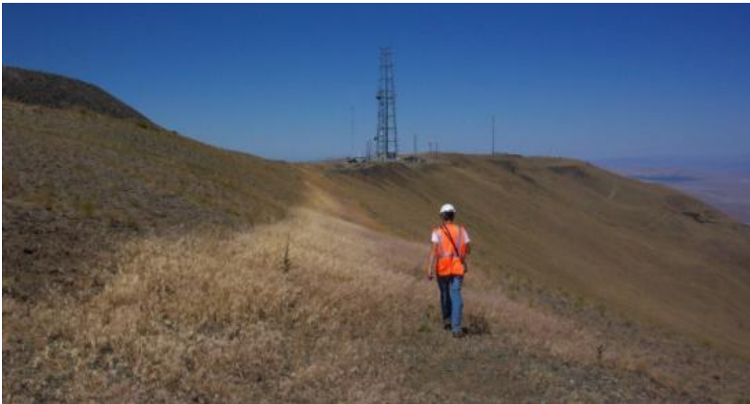
Figure 2.9. Unit 4: Linear Area Associated with Removal of Overhead Powerline and New Underground Power Service
