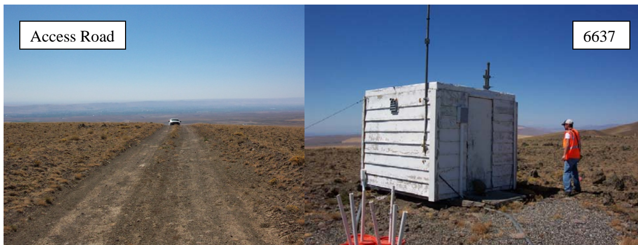
Figure 2.12. Example of Road and Parking/Access to Communication Facilities in Unit 6
