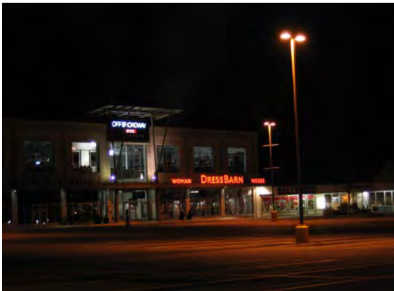
Figure 2.2. Original HPS Luminaires
