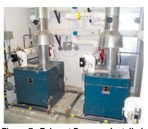
Figure 7. Exhaust Dampers Installed
