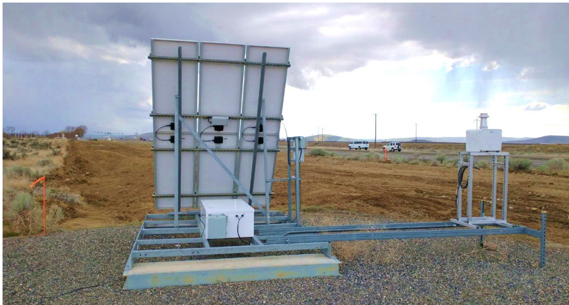
Figure 3.2. PNL-1 after Surface Soil Grading in Preparation for Waterline Improvements
