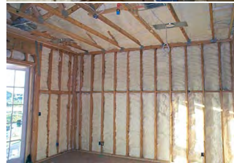
(1) Batt insulation. (2) Blown-in insulation. (3) Foamed-In-Place. (Photo source: Sam Garst) (4) Here, spray foam is applied along the underside of the roof deck to provide a conditioned and non-vented attic space for ducts and air handlers.
