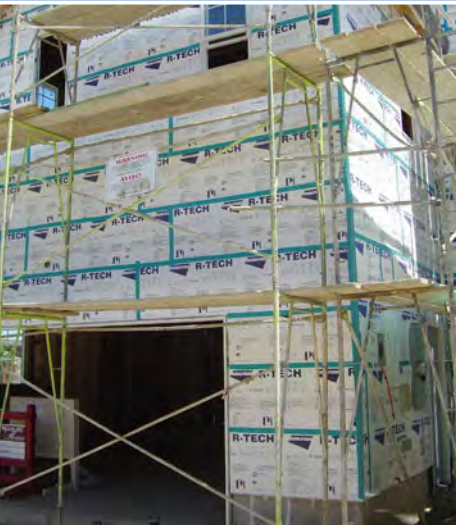
Treasure Homes of Sacramento installs rigid foam under stucco siding to serve as an insulation layer and exterior vapor barrier.
