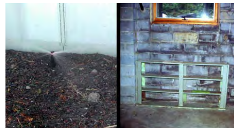
This sprinkler was placed too close to the house's foundation wall. Moisture seeped through the concrete block causing water stains and mold inside. (Photo source: EPA; photo by Terry Brennan)
