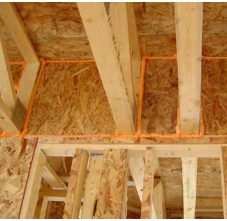
In this figure, OSB and foam form the air barriers to isolate the garage from living space.
