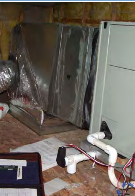
The air handler is located inside the conditioned attic.
