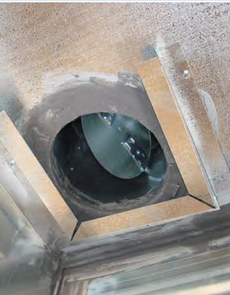
A mechanical damper on the fresh air intake lets fresh air into the air handler box when needed to provide fresh supply air for the HVAC system.
