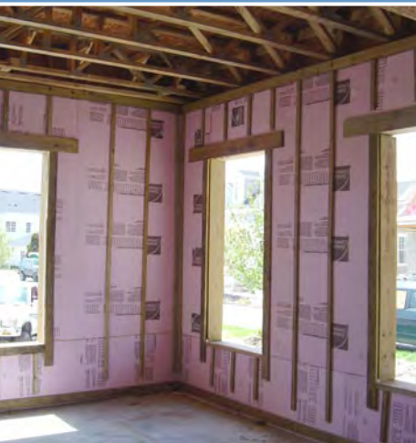
Masonry walls are insulated with interior rigid insulation.
