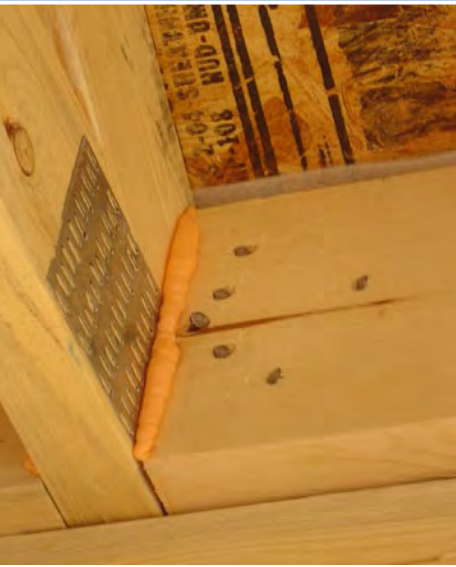
The intersection of walls, ceilings, and attic trusses must be sealed in non-vented attics. This example uses gaskets and canned spray foam for the seal.
