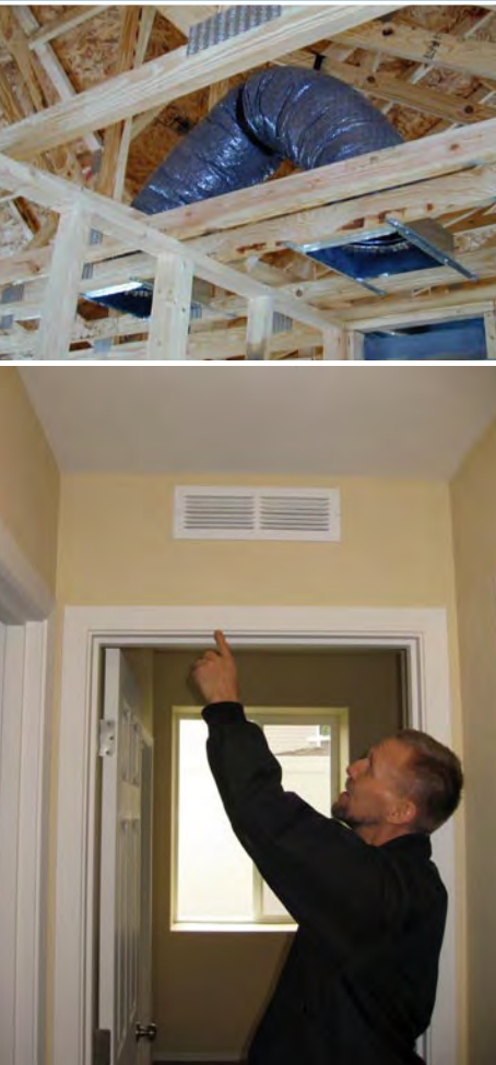
(top) Installing jump ducts from room to room is one way to balance pressures. (Photo source: IBACOS)
