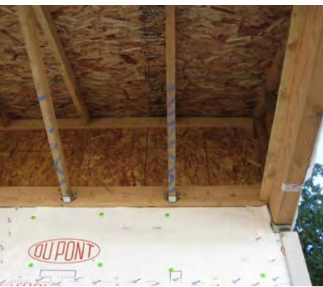
Framing is sequenced to install an air barrier between the porch roof cavity and conditioned space.
