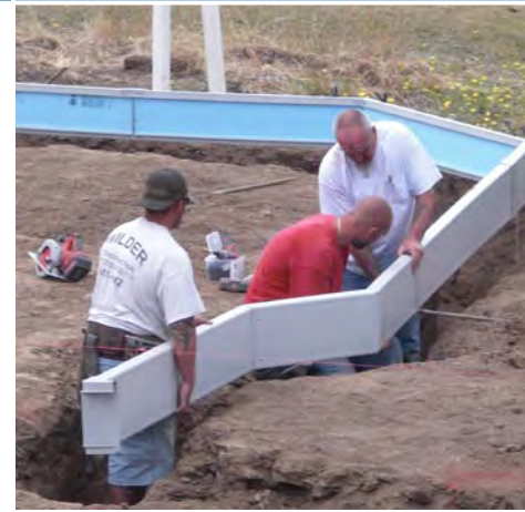
Davis Energy Group of the CARB Building America team developed a new method for insulating slab perimeters that is ideal for extremely hot climates and mixed dry climates. The method, which is still being tested, uses termiticide-treated rigid foam insulation encased in PVC as the form for the concrete foundation.
