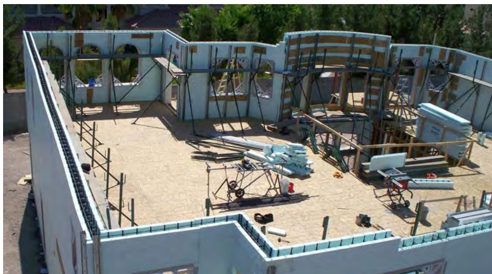
Insulated concrete form (ICF) walls form a solid thermal boundary for the NextGen 2009 home in Las Vegas. (Photo source: iShow.com, Inc.)
