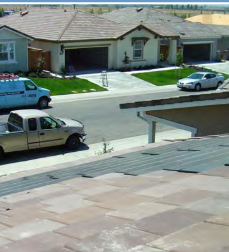
Powerlight integrated solar roof tiles blend in with surrounding roof tiles to provide 2.4 kw of clean, quiet energy.
