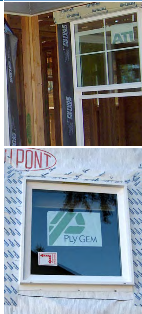
(top) Windows should be flashed in accordance with ASTM E2112-07.
