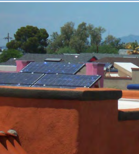
The southwestern architecture of John Wesley Miller's Armory Park del Sol urban infill project cleverly hides the rooftop photovoltaic and solar water heating panels from passersby.
