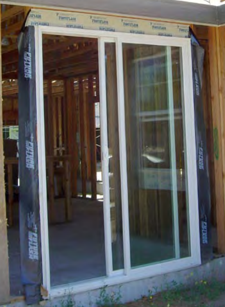
Flashing, gaskets, and caulk are used to air seal around penetrations in the building envelope under brick, stucco, and lap siding exteriors.
