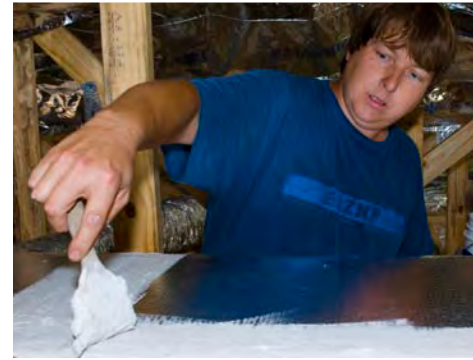
Mastic provides the most reliable duct sealing method. Ducts should be located in conditioned space. (Photo source: BAIHP)
