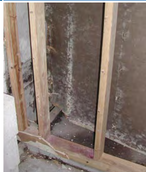
When moisture is trapped inside walls, mold can grow unchecked causing damage to the walls and health impacts for the occupants. (Photo source: EPA; photo by Terry Brennan)
