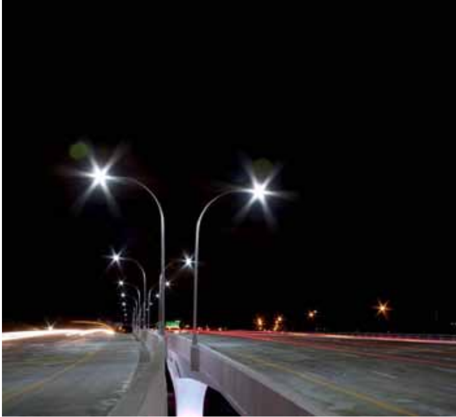
Figure 2.1. Luminaires installed on the I-35W Bridge.
