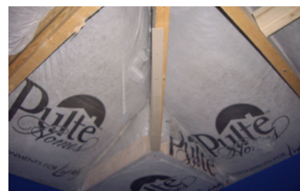
Figure 16.4. Insulation in non-vented attics is applied directly under roof sheathing. (Photo courtesy of Pulte Homes)
