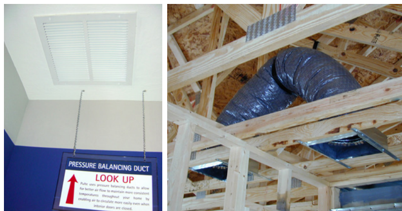
Figure 26.1. Jump ducts
