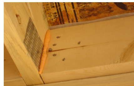
Figure 16.4. Insulation in non-vented attics is applied directly under roof sheathing. (Photo courtesy of Pulte Homes)
