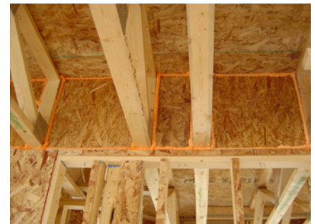
Figure 16.1. In this figure, OSB and foam form the air barriers to isolate the garage from living space.
