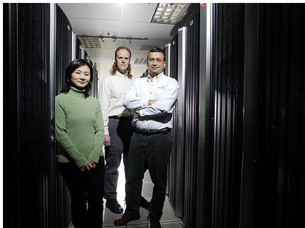
Figure 1.2. The 163-TFlop Chinook supercomputer is housed in the MSC.
