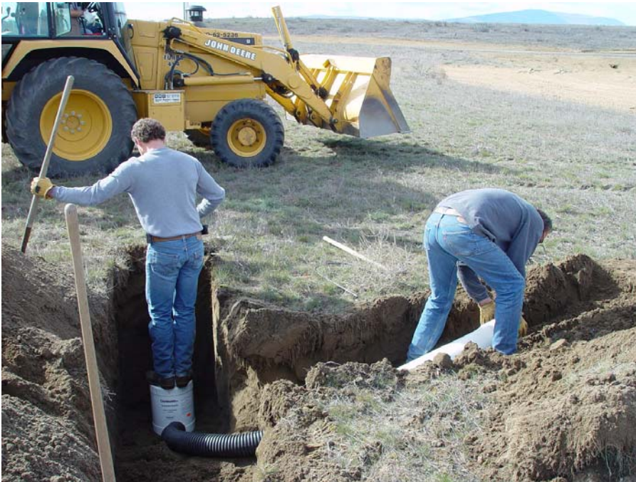
Figure 1. Construction of the Artificial Burrows
