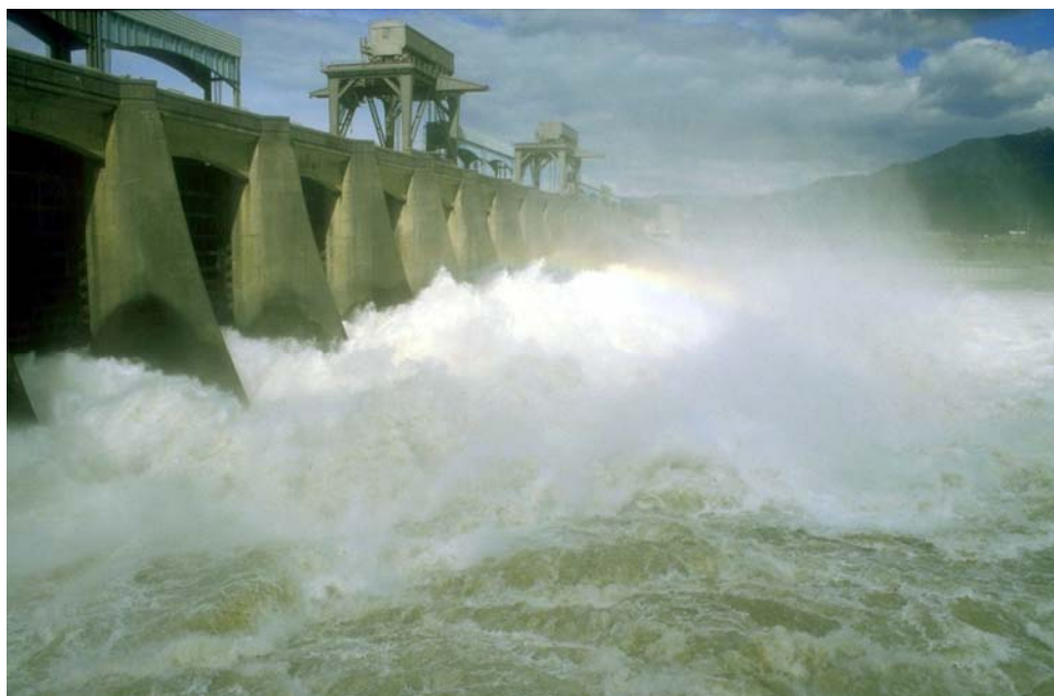
Figure 4.2. Spill discharge for fish passage at Bonneville Dam.
