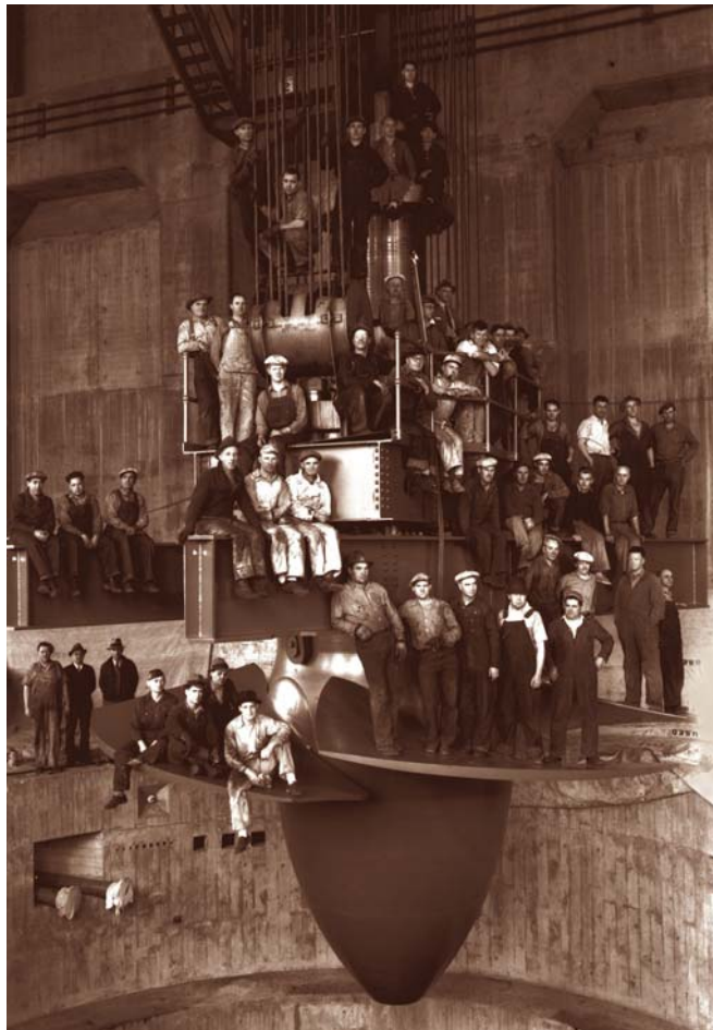
Figure 4.1. One of the original Kaplan turbine runners installed in the later 1930s at the Bonneville Dam first powerhouse. This runner is typical of those installed at most dams below Chief Joseph Dam on the mainstem Columbia River.
