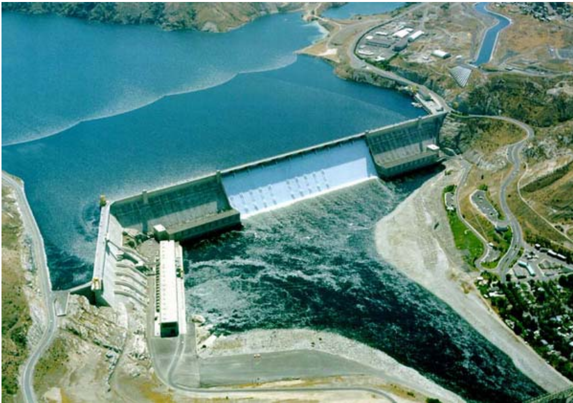
Figure 2.1. Grand Coulee Dam, Washington. The Pump-Generation Plant is shown in the upper right of the photo just above the left powerhouse.
