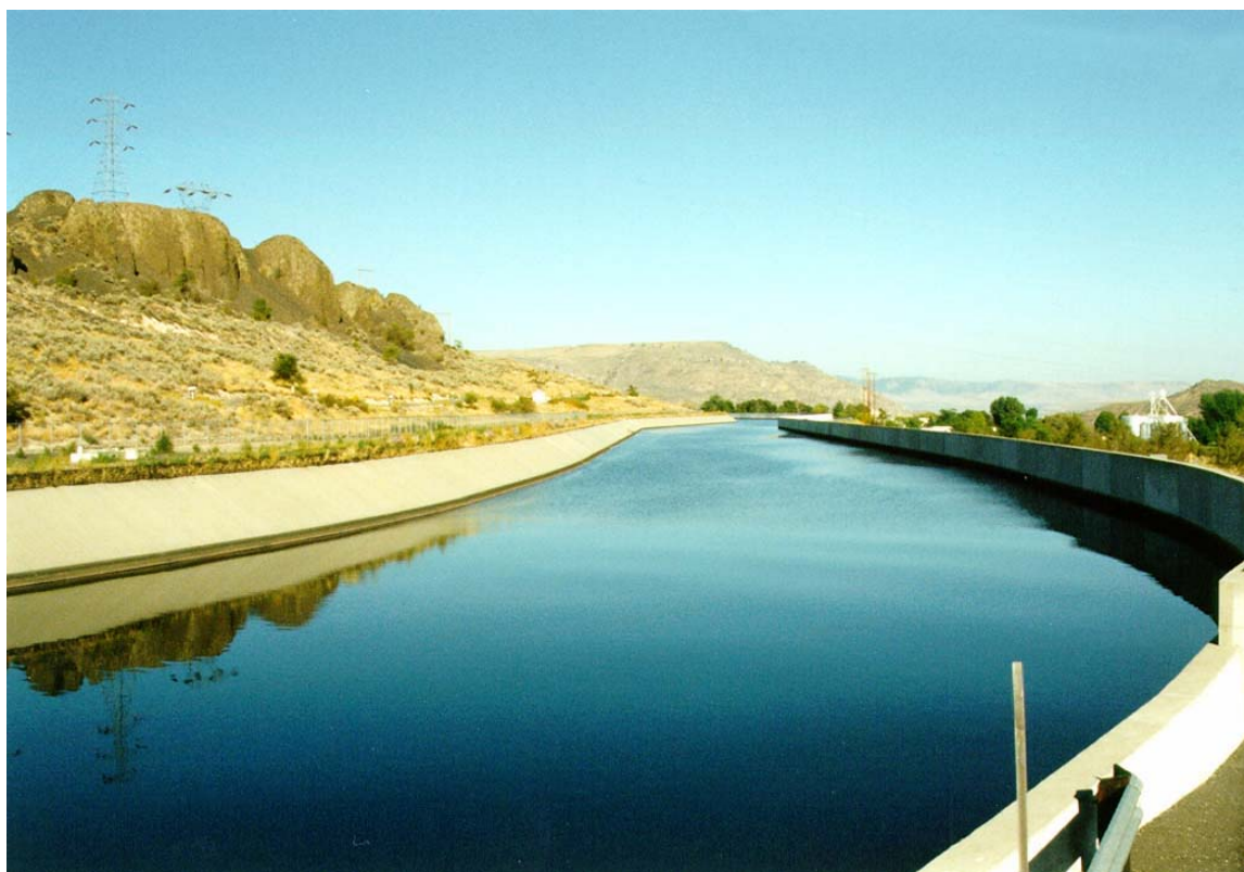
Figure 2.2. Canal carrying water from Lake Roosevelt through the pump-generating units to Banks Lake.
