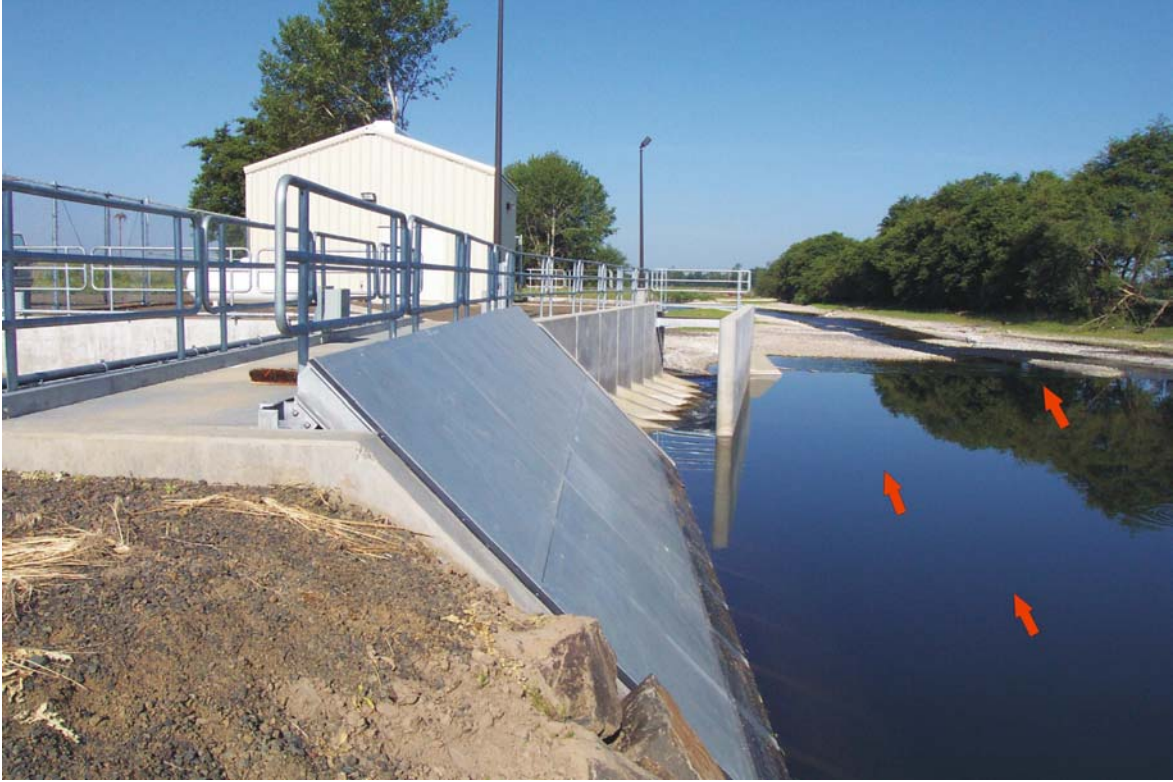
Figure 1.3. Garden City/Lowden II Fish Screens. The red arrows show the direction of water flow.
