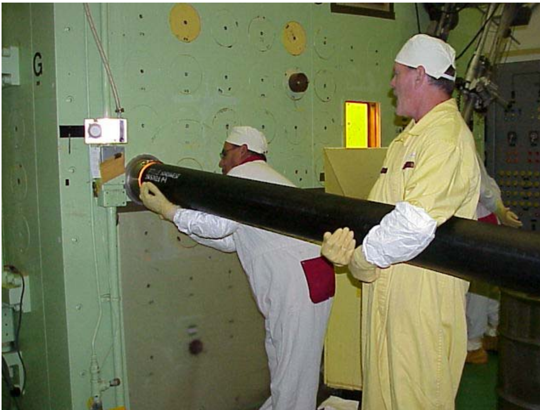
Figure 5.2. Workers inserting the traverse pipe into a port in G Cell.
