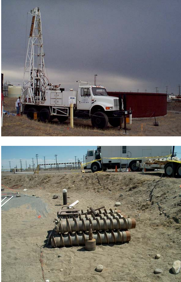
Figure 8. Drilling of the Mock Tank Wells for FY 2001 Using Hollow-Stem Auger Methods. Access to locations around the tank for drilling was difficult due to pre-existing well casings and limited maneuvering space. The preexisting casings were cut to near ground level to improve access.
