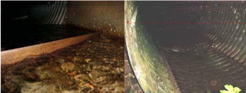
Figure 6. Photo of baffle and wier configurations inside Parish Creek culvert.
