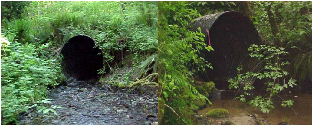
Figure 5. Parish Creek culvert inlet (left photo) and outlet (right photo), June 2001.
