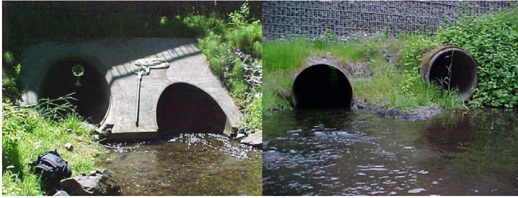
Figure 2. Dogfish Creek culvert inlet (left photo) and outlet (right photo), June 2001.
