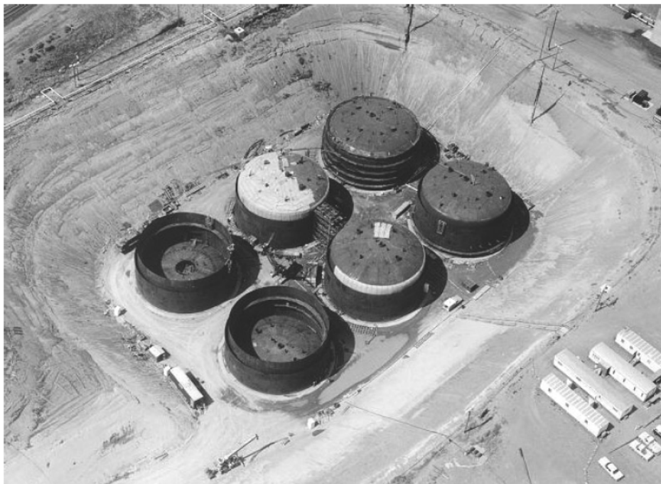
Figure 1.1. Double-Shell Tank Farm under Construction, circa 1980
