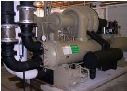
Typical Centrifugal Chiller
